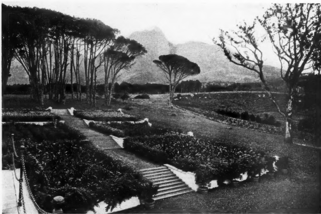
GROOTE SCHUUR: VIEW FROM REAR OF HOUSE
