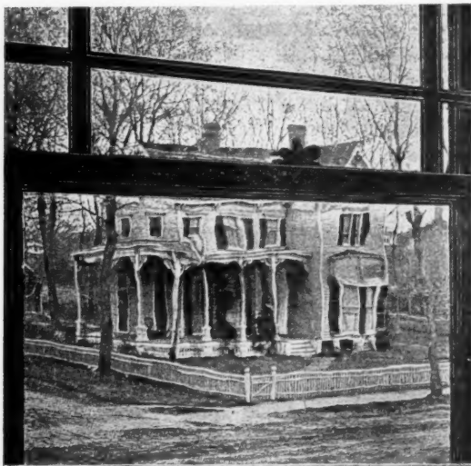
THE DISTORTED VISION GIVEN BY BADLY FLAT-TENSIONED WINDOW GLASS
