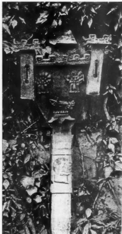
LEAD RAINWATER HEAD, HADDON HALL
