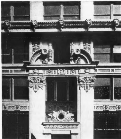
DETAIL OF HEARST BUILDING, CHICAGO, ILL.
