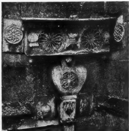
LEAD RAINWATER HEAD, HADDON HALL
