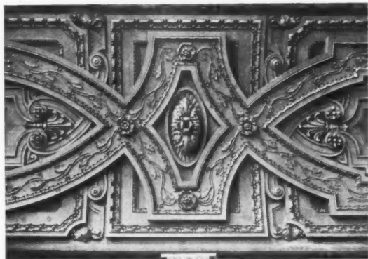
MAIN LOGGIA CEILING PANEL IN STATE EDUCATIONAL BUILDING, ALBANY, N. Y.
