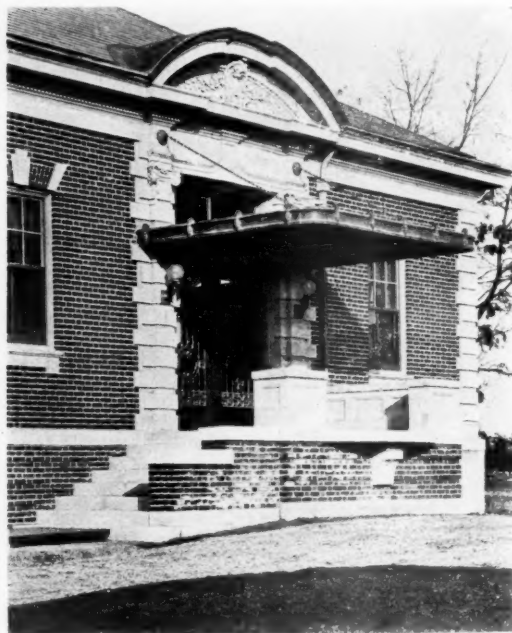
AMBULANCE ENTRANCE, BROCKTON HOSPITAL, BROCKTON, MASS.
