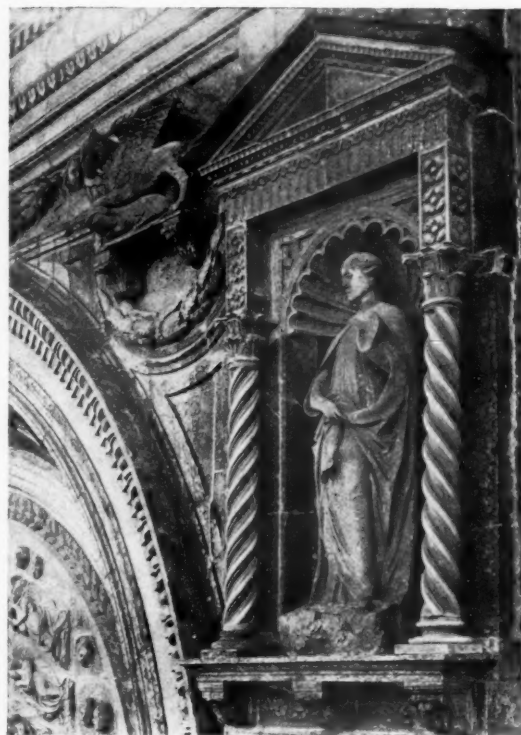
EXTERIOR DETAIL, CHURCH OF S. BERNARDINO, PERUGIA
