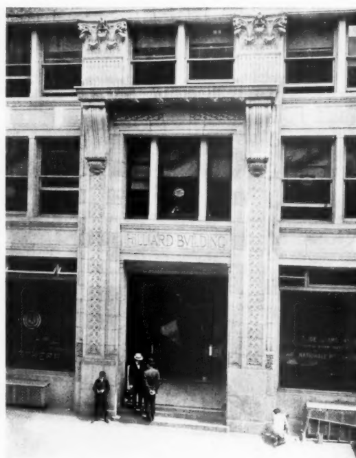
DETAIL OF ENTRANCE THE HILLIARD BUILDING MESSRS. HOWELLS & STOKES, ARCHITECTS
