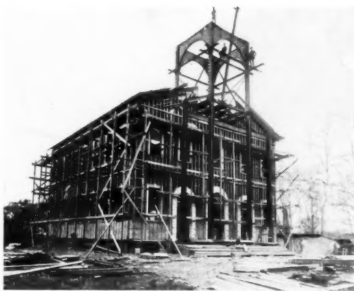
VIEW DURING CONSTRUCTION
