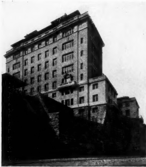
HOSPITAL BUILDING, ROCKEFELLER INSTITUTE FOR MEDICAL RESEARCH
