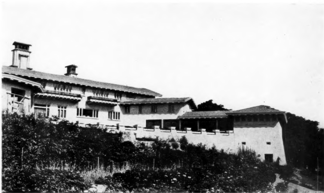
SOUTH VIEW OF NORTH WING
