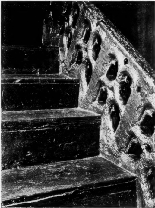
STAIRCASE WITH STONE BALUSTRADE DOWNHOLLAND HALL, NEAR ORMSKIRK
