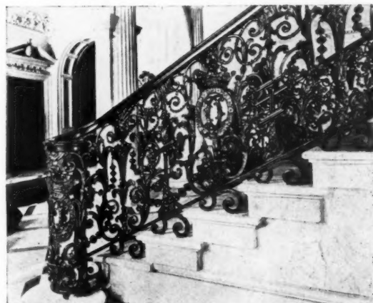
IRON BALUSTRADE, CHESTERFIELD HOUSE, LONDON
