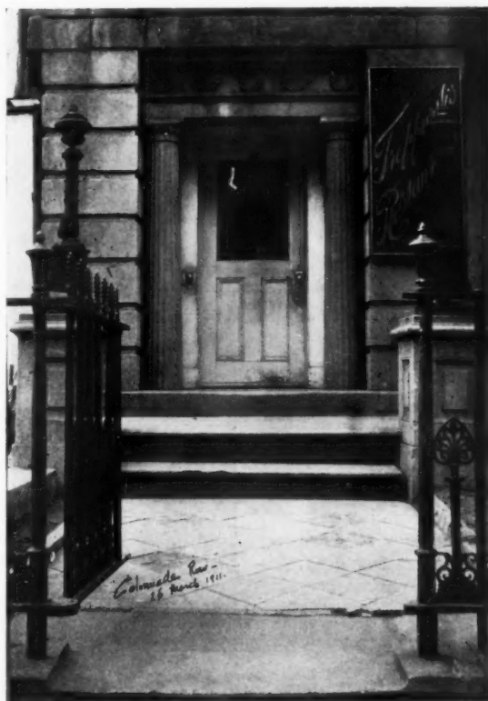
DETAIL OF ENTRANCE
