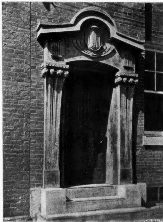
ENTRANCE DETAIL, OFFICE BUILDING, FOR BROWN BROS. MANUFACTURING CO. MESSRS. HILL & WOLTERS DORF, Architects The door frame is of cast iron
