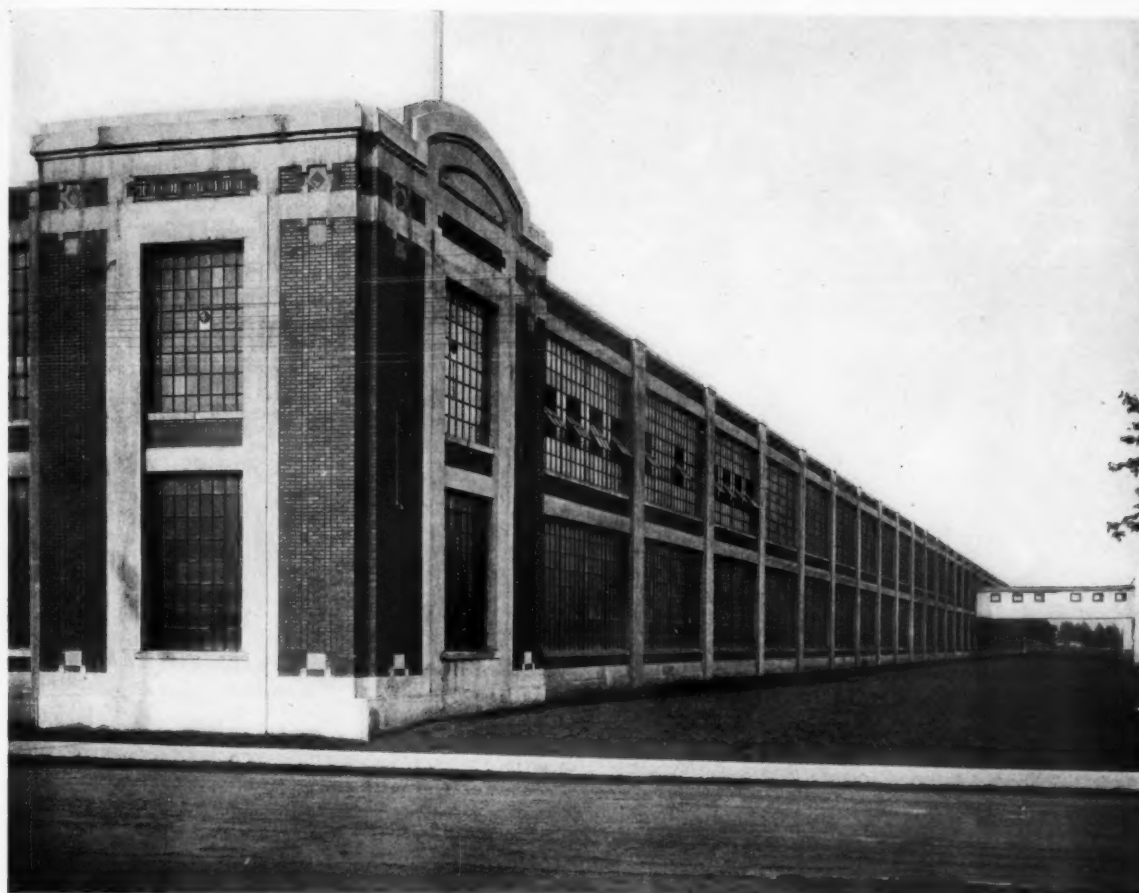
MAIN FACTORY BUILDING, HUDSON MOTOR CO., DETROIT, MICH. MR. ALBERT KAHN, Architect . MR. ERNEST WILBY, Associate
