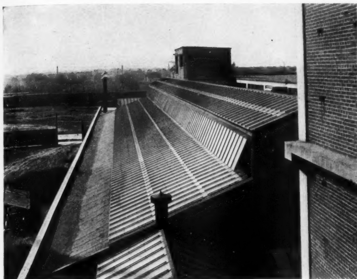
ROOF OF MOTOR TRUCK SHOP, PACKARD MOTOR CAR CO., DETROIT, MICH. MR. ALBERT KAHN, Architect . MR. ERNEST WILBY, Associate This skylighting affords a maximum of light
