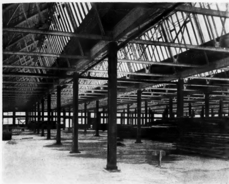
INTERIOR OF FACTORY FOR MESSRS. BLAKE & JOHNSON CO., WATERTOWN, CONN. MESSRS. GRIGGS & HUNT, Architects
