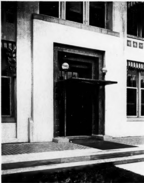
ENTRANCE TO ADMINISTRATION BUILDING, HUDSON MOTOR CO., DETROIT, MICH.
