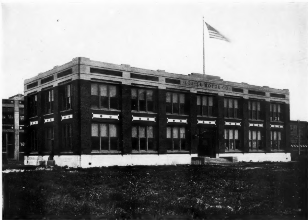
ADMINISTRATION BUILDING, LOZIER MOTOR CO., DETROIT, MICH. MR. ALBERT KAHN, Architect ; MR. ERNEST WILBY, Associate
