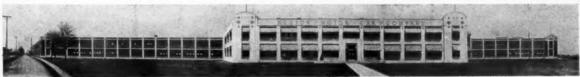
HUDSON MOTOR CO.'S PLANT, DETROIT, MICH. MR. ALBERT KAHN, Architect . MR. ERNEST WILBY, Associate
