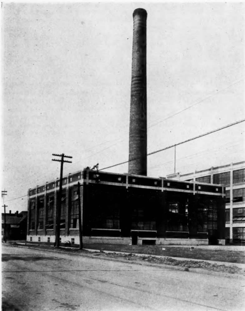
POWER BUILDING, MESSRS. DODGE BROS., DETROIT, MICH. MR. ALBERT KAHN, Architect. MR. ERNEST WILBY, Associate
