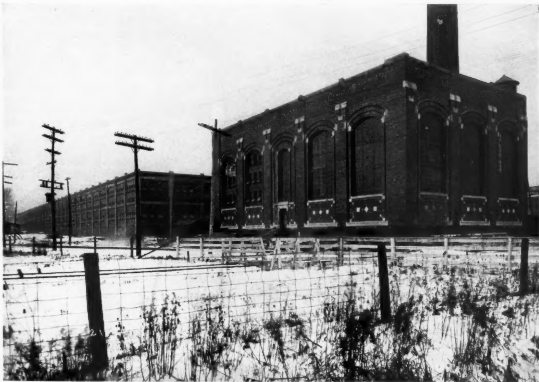
POWER HOUSE AND MAIN BUILDING, LOZIER MOTOR CO., DETROIT, MICH. MR. ALBERT KAHN, Architect. MR. ERNEST WILBY, Associate
