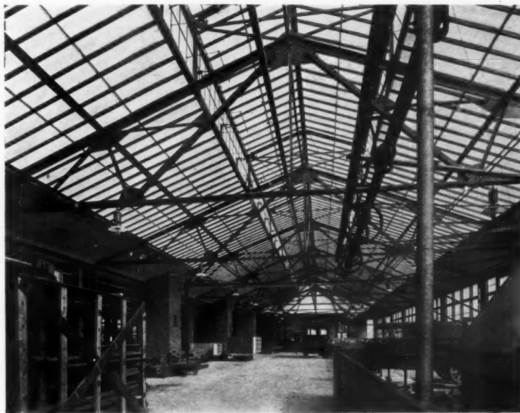
INTERIOR OF MOTOR TRUCK SHOP, PACKARD MOTOR CAR CO., DETROIT, MICH. MR. ALBERT KAHN, Architect . MR. ERNEST WILBY, Associate
