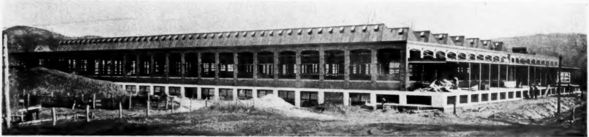
FACTORY BUILDING FOR MESSRS. BLAKE & JOHNSON CO., WATERTOWN, CONN. MESSRS. GRIGGS & HUNT, Architects
