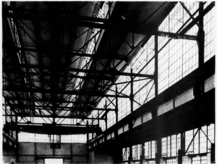
FORGE SHOP, PACKARD MOTOR CAR CO., DETROIT, MICH. MR. ALBERT KAHN, Architect . MR. ERNEST WILBY, Associate Note method of crane support.
