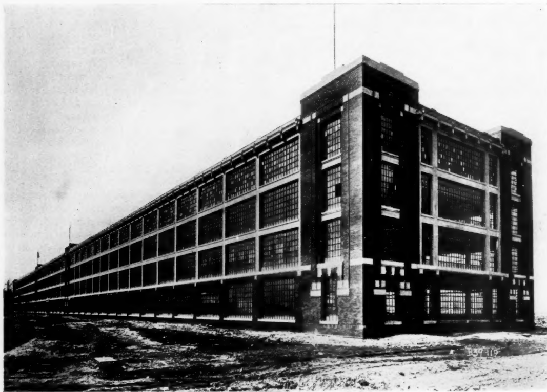
ONE OF A GROUP OF FACTORY BUILDINGS FOR FORD MOTOR CO., DETROIT, MICH.
