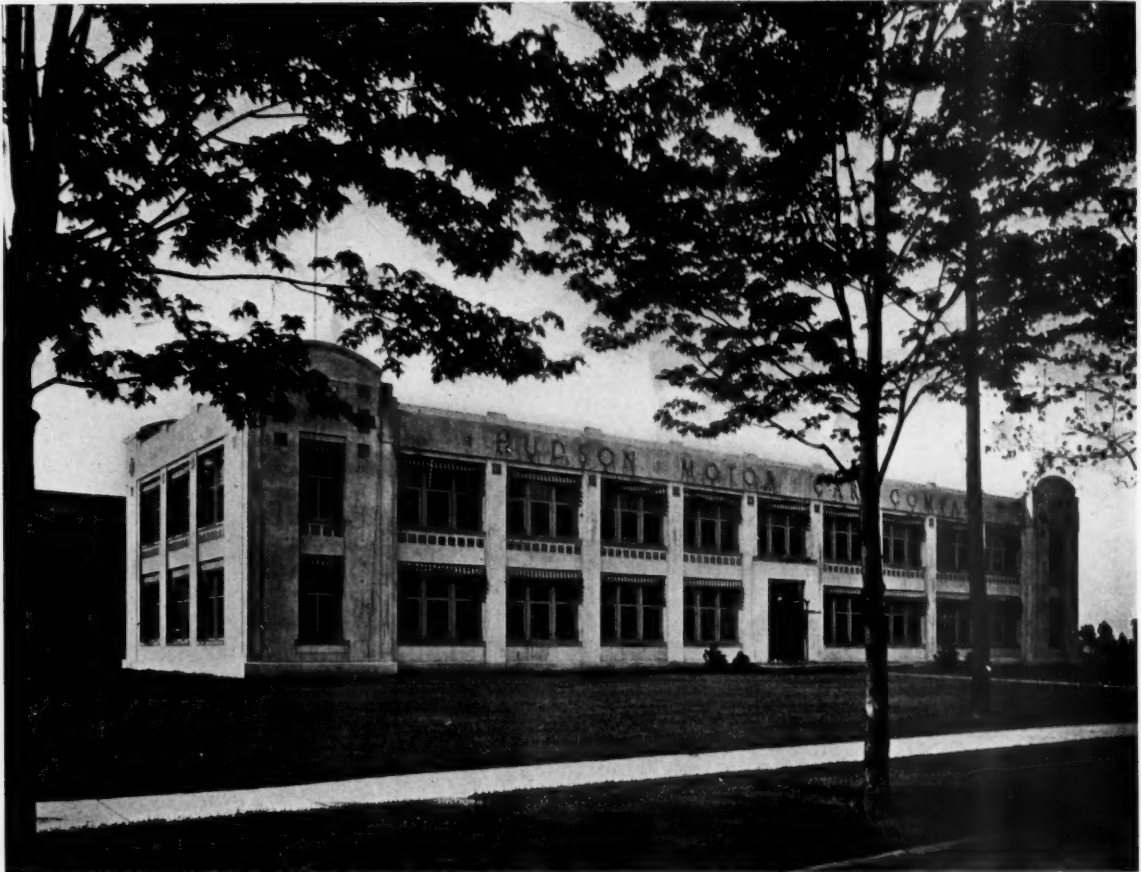
ADMINISTRATION BUILDING, HUDSON MOTOR CO., DETROIT, MICH.
