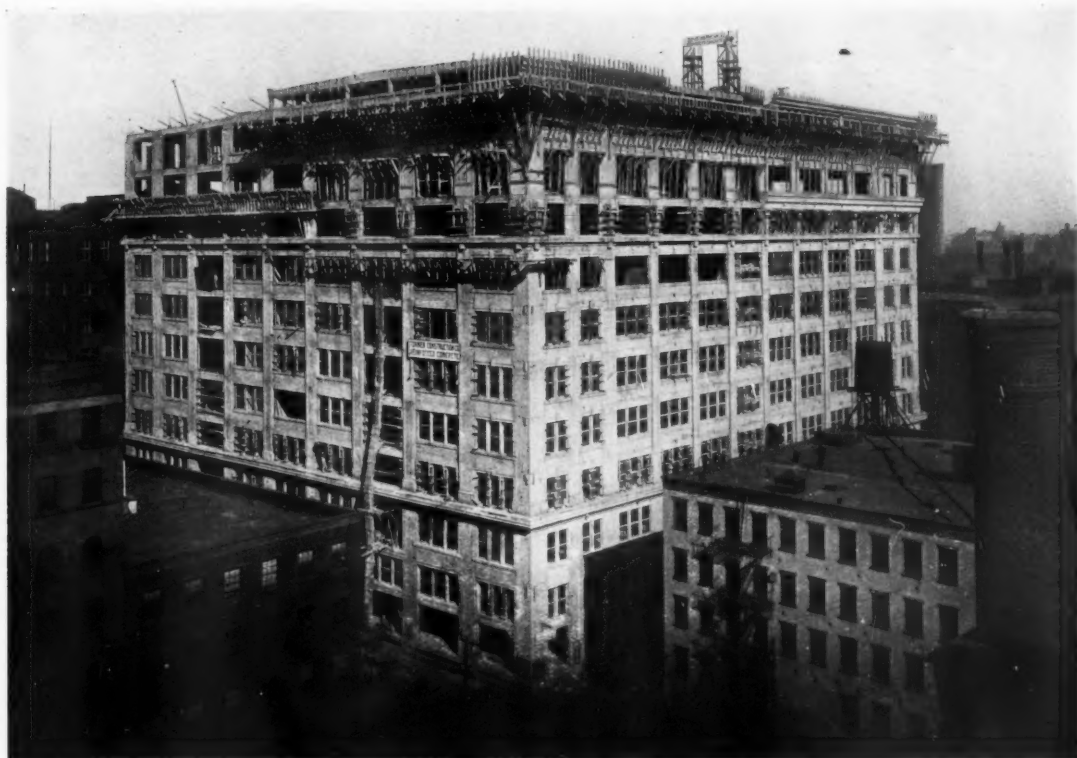
VIEW OF UPPER STORIES DURING CONSTRUCTION
