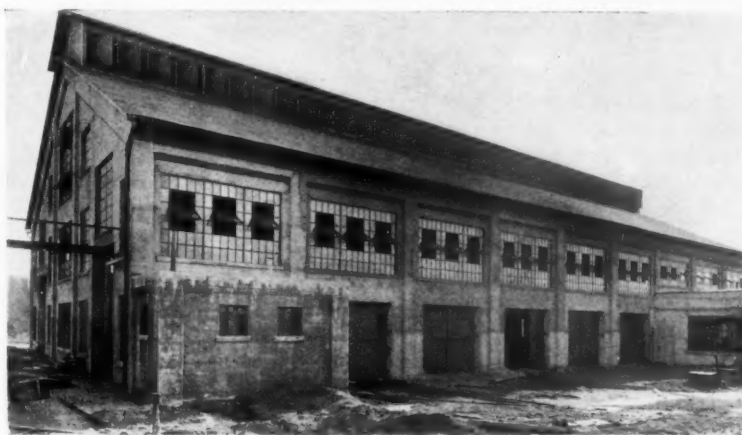
FORGE SHOP, MESSRS. BILLINGS & SPENCER CO. MESSRS. FORD, BUCK & SHELTON, Architects
