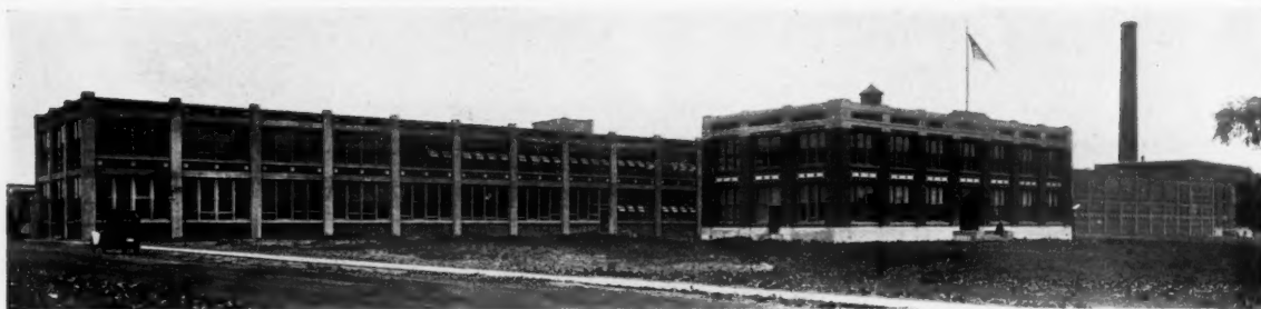
GENERAL VIEW, PLANT OF THE LOZIER MOTOR CO., DETROIT, MICH. MR. ALBERT KAHN, Architect . MR. ERNEST WILBY, Associate
