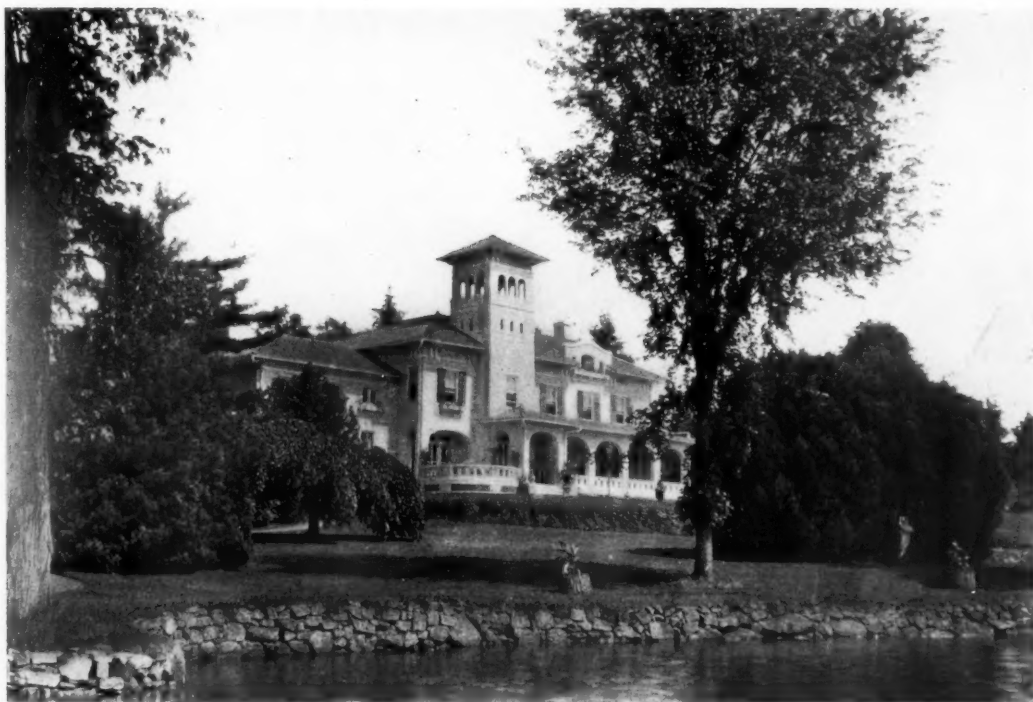
HOUSE AFTER ALTERATIONS
