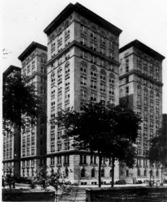
THE TURIN APARTMENTS, NEW YORK ALBERT J. BODKER, Architect From Architecture
