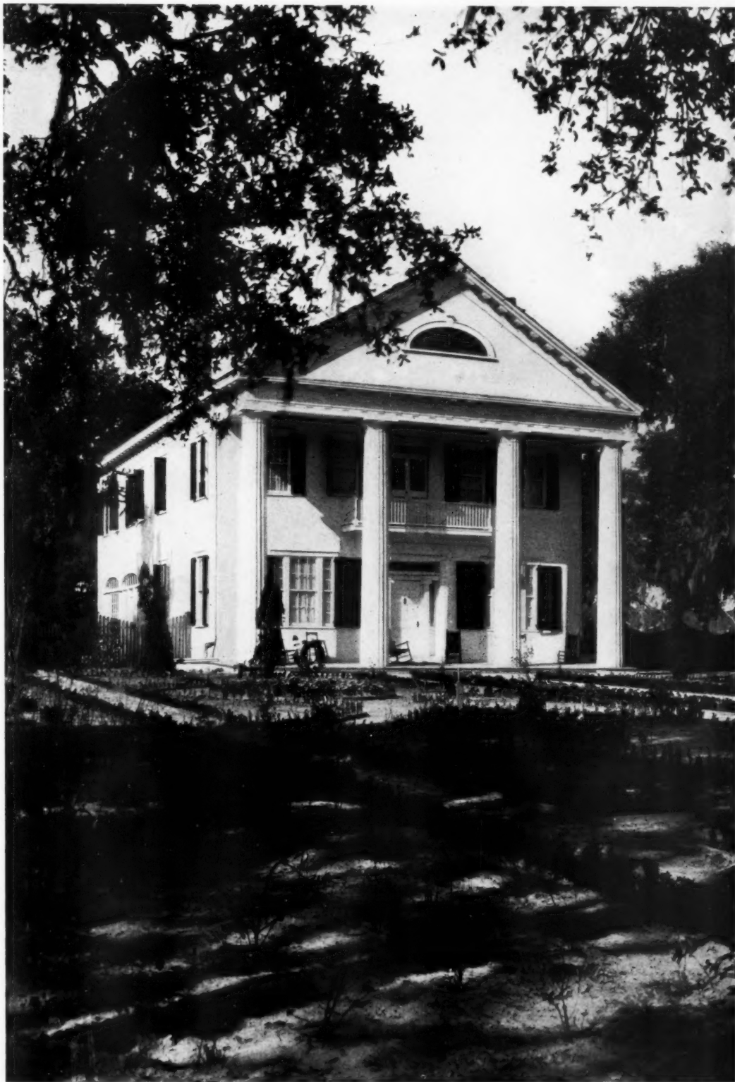
HOUSE BEFORE ALTERATIONS
