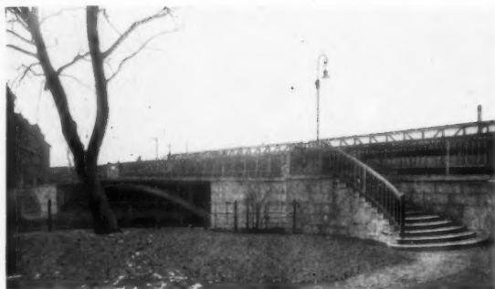
KOETHNER BRIDGE, BERLIN A. KOENIG, Architect
