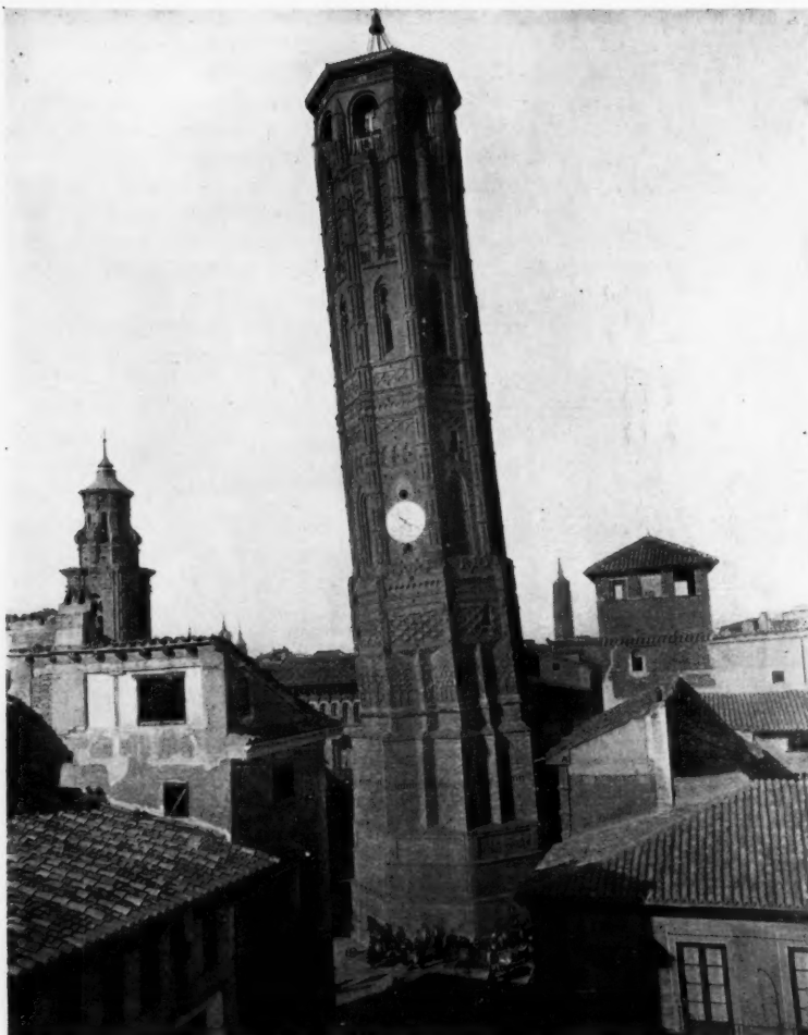
LEANING TOWER, SARAGOSSA, RECENTLY DEMOLISHED
