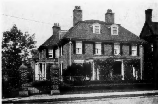
HOUSE IN PITTSBURGH GEORGE ORTH & BROTHER, Architects
