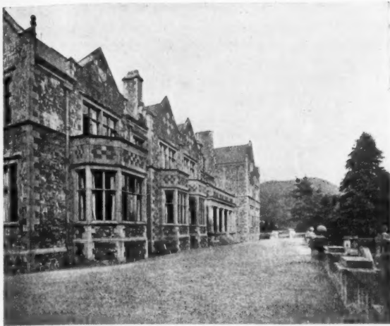
Terrace, Grizedale Hall, Lancashire, Eng. Walker, Carter & Walker, Architects (From The International Studio )
