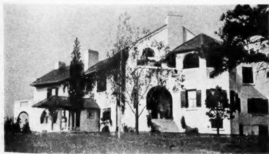
HOUSE FOR CHARLES RICHMAN, ESQ., WOODBURY, N. Y. ALFRED HOPKINS, Architect
