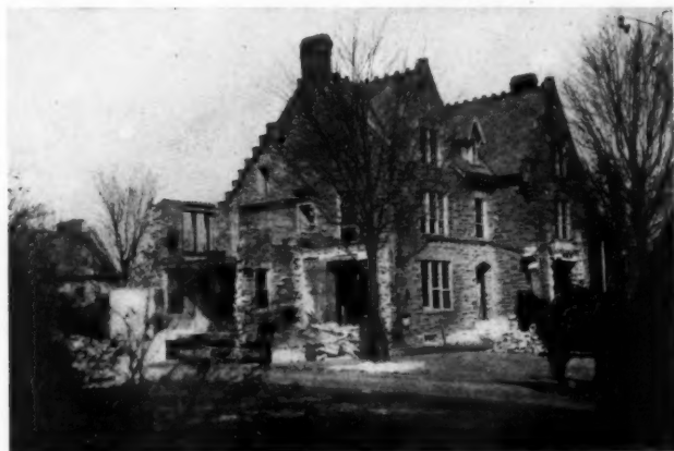
THE HOUSE BEFORE ALTERATIONS
