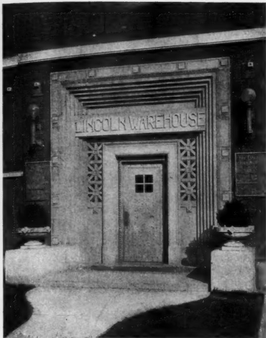
Fig. 6, Entrance: The Lincoln Fireproof Storage Warehouse, Chicago, Ill. Ottenheimer, Stern & Reichert, Architects (From The Architectural Record )
