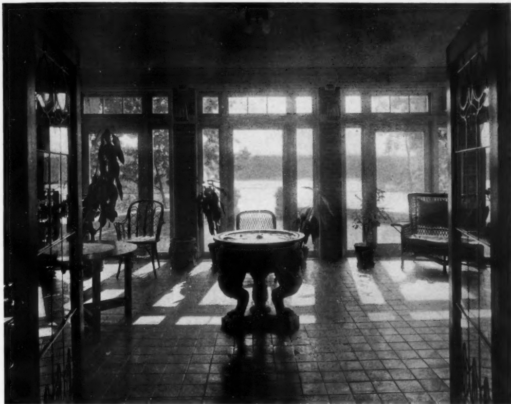
Sunroom, on main axis of entrance hall, looking towards terrace and lake. Walls of tapestry brick. Floors, moss-green dull-glaze tile. Doors of mahogany with leaded plate glass. Fountain of Italian (Carrara) marble.
