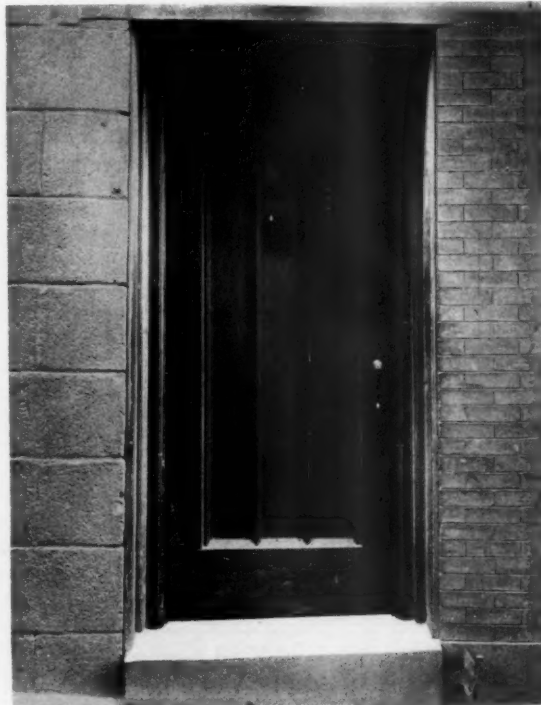
ENTRANCE, 16 SOMERSET STREET
