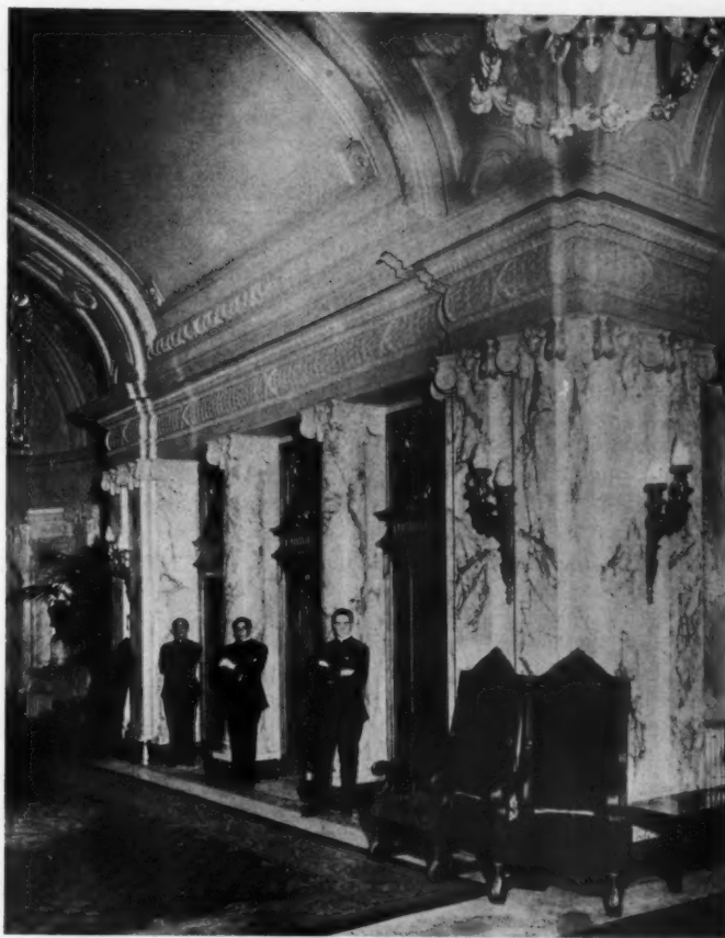
THE ELEVATOR ENTRANCES—HOTEL RECTOR, NEW YORK
