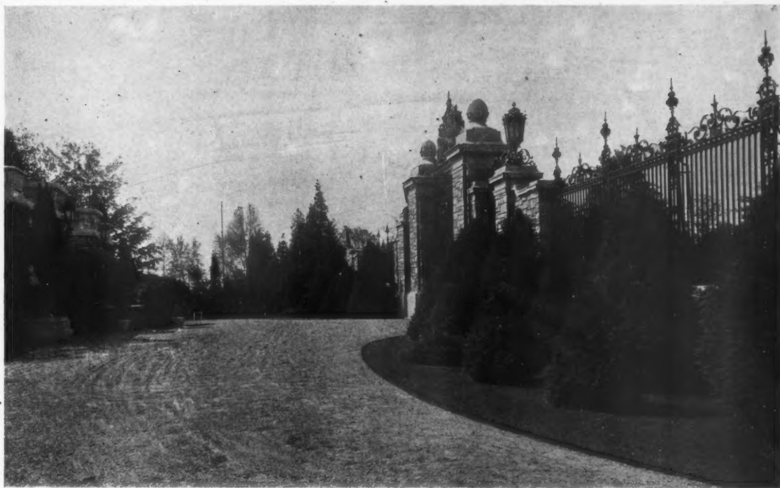
PLATE I—ENTRANCE GATES. EXEDRA FOUNTAIN ON THE LEFT. THE VIEW IS TAKEN LOOKING SOUTH AND SHOWS THE BEGINNING OF THE NEW ENTRANCE DRIVEWAY. THE FLAGPOLE AT THE END OF THE TENNIS COURT IS SEEN IN THE DISTANCE
