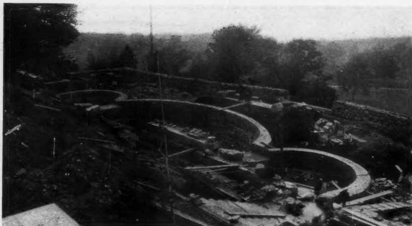
FIG. E—VIEW OF SWIMMING POOL TERRACE DURING CONSTRUCTION. THE EFFECT JUST AFTER THE PLANTING WAS DONE IS SHOWN IN CUT Q
