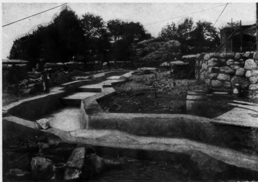
FIG. I—THE BROOK GARDEN UNDER CONSTRUCTION. THE CONCRETE WALLS WERE COVERED WITH ROCKS AND THE BOTTOM WITH PEBBLES
