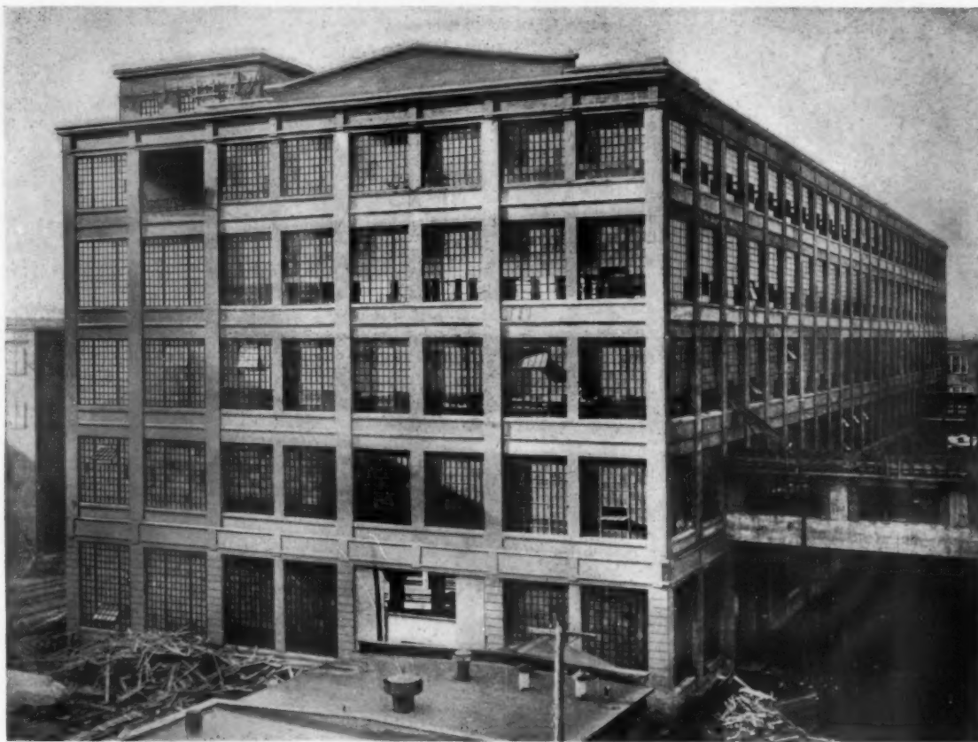
Building No. 42, General Electric, Schenectady, N. Y., equipped throughout with over 50,000 square feet of United Steel Sash.
