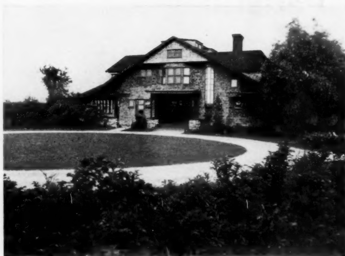
Residence of F. I. Cooper, Mayland, Mass. Cooper & Bailey, Architects, Boston Covered with Winthrop Asphalt Shingles
