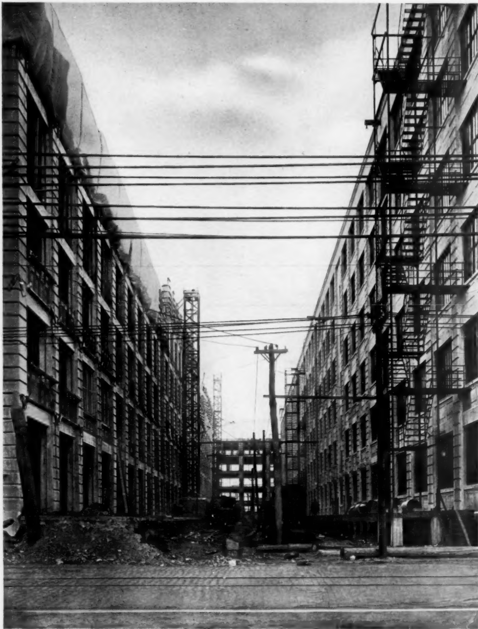
VIEW BETWEEN MODEL FACTORIES 3 and 4. BUSH TERMINAL CO. FACTORIES, 36th St., Brooklyn, N. Y. Factory No. 3, 600' x 75' Factory No. 4, 750' x 75' Each Six Stories and Basement. William Higginson, Architect.
