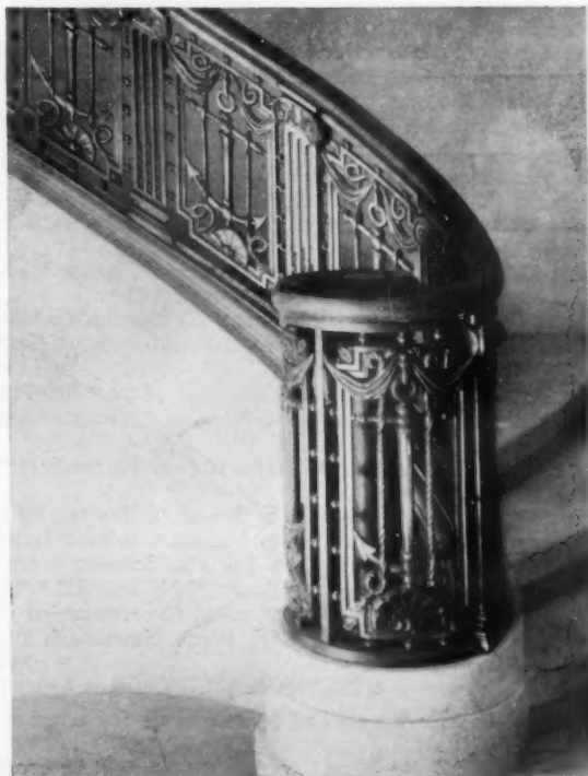
STAIR RAIL U. S. CUSTOM HOUSE, NEW YORK CASS GILBERT, ARCHITECT
