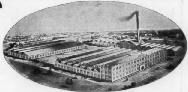
American Ball Bearing Co., Cleveland, O. Covered with 100,000 square feet of J-M Asbestos Roofing
