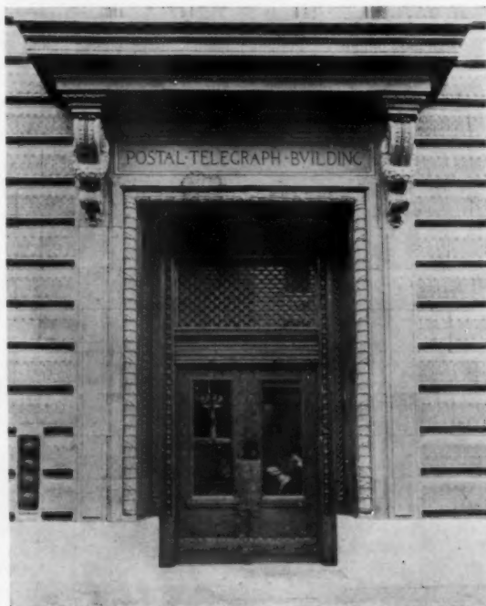
BRONZE ENTRANCE DOORS POSTAL TELEGRAPH BLDG., SAN FRANCISCO. Lewis P. Hobart, Architect.
