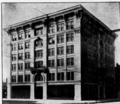
Vermont Building, Salt Lake City. Metal Lumber used throughout for Interior Construction. Monroe & Schaub, Architects.
