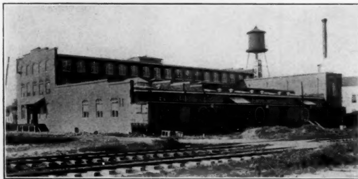
New factory building of the Hackney Wagon Co., at Wilson, N. C., covered with 150 squares of "TARGET AND ARROW" tin in September, 1909, by R. E. Hagan, roofer, Wilson, N. C.
