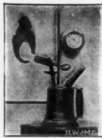
In this test the flame of a powerful blowtorch was placed within two inches of J-M Asbestos Roofing. At the end of fifty minutes the roofing was not burned or injured, being only slightly blackened with smoke.
