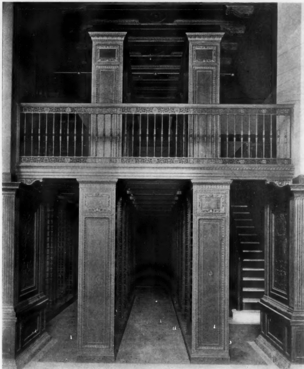
View of typical stack bay in the Technical Science Reading Room of the New York Public Library, Carrere & Hastings, Architects
