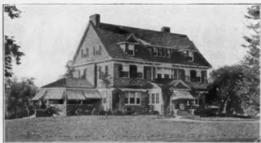
RESIDENCE AT SCARSDALE, N. Y.
