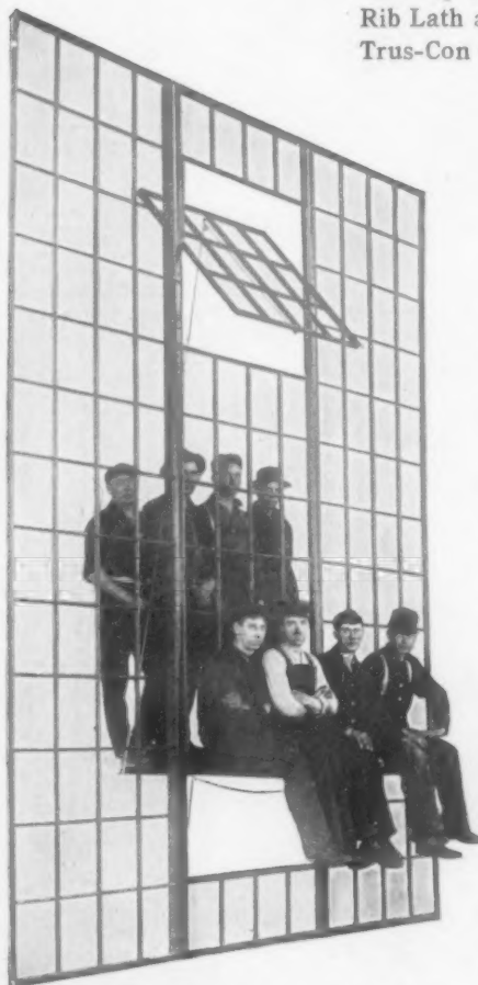
Remarkable Strength of United Steel Sash, Eight Men Balanced on Ventilator.
