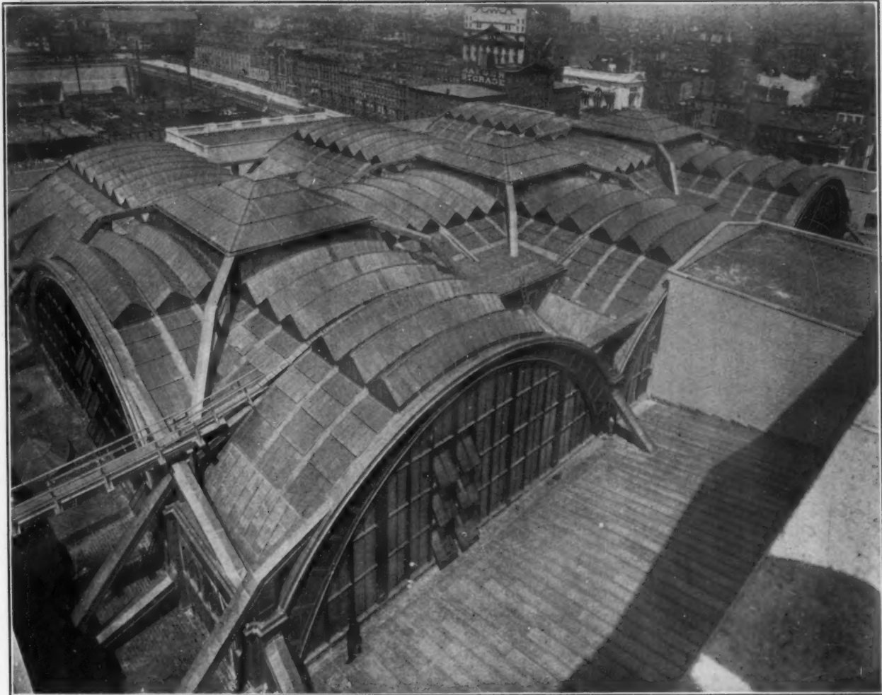
SKYLIGHTS OVER THE PENNSYLVANIA TERMINAL CONCOURSE
