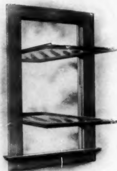
Showing Upper Sash Lowered and Reversed for Cleaning.
