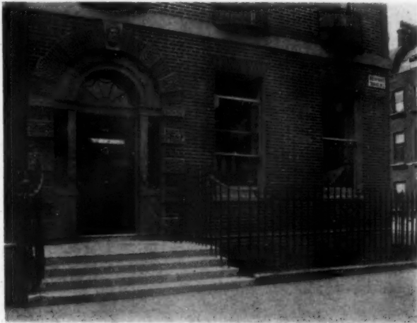
ENTRANCE, THE SOCIETY OF ARCHITECTS, 28 BEDFORD SQUARE, LONDON
