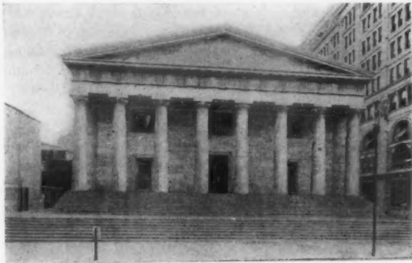
CUSTOM HOUSE, PHILADELPHIA, PA., 1817-1824 BENJAMIN H. LATROBE, Architect.
