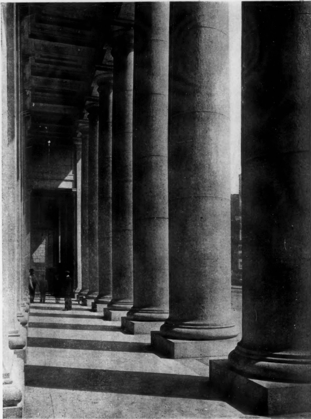
THE COLONNADE ON SEVENTH AVENUE FRONT, LOOKING NORTH
