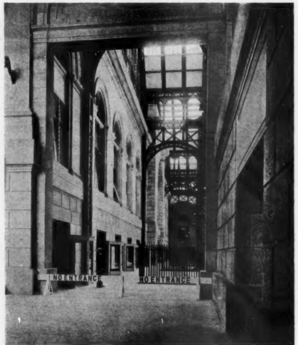
VIEW SOUTH FROM TRAFFIC-WAY ALONG EAST SIDE OF CONCOURSE. THIS VIEW SUGGESTS THE DIFFICULTIES TO BE ENCOUNTERED IN PRESERVING THE SCALE BETWEEN STEEL AND STONE ARCHITECTURE
