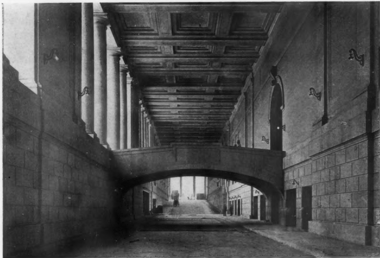
THE TRAFFIC WAY, THIRTY-THIRD STREET SIDE, LOOKING TOWARDS SEVENTH AVENUE
