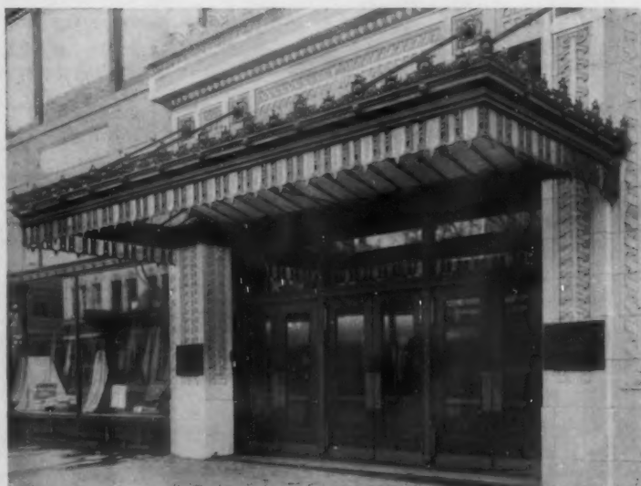
CANOPY, BAILLARGEON BUILDING, SEATTLE Saunders & Lawton, Architects
