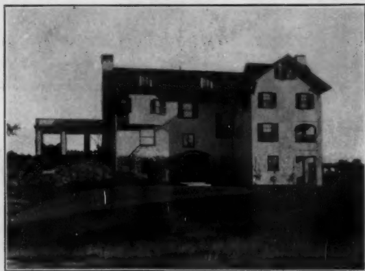
KELSEY HEATED RESIDENCE, GREENWICH, CONNECTICUT Kirby, Pettit & Green, Architects, New York
