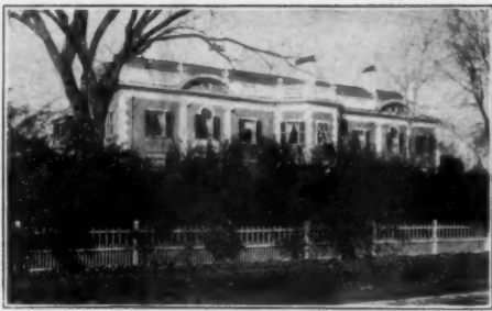
RESIDENCE OF HON. GEORGE VON L. MEYER, Secretary of the Navy, Hamilton, Mass. Little & Browne, Architects, Boston. Stained with No. 403 Italian Pink Cement Stain.
