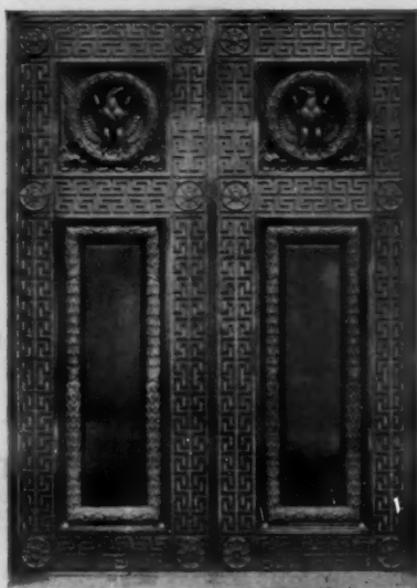
BRONZE ENTRANCE DOORS ROCHESTER TRUST AND SAFE DEPOSIT CO. YORK & SAWYER, ARCHITECTS.
