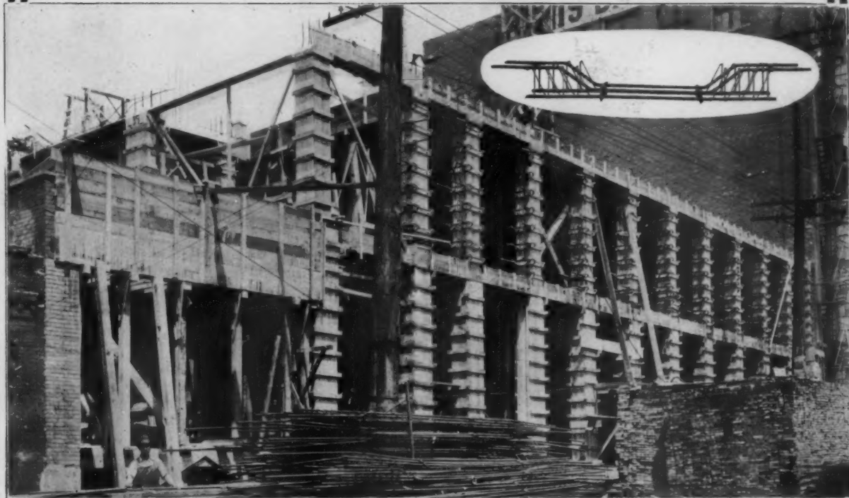
Bemis Bros Bag Co., St. Louis, Mo Corrbars Units—Shop Fabricated Reinforcement JAMES BLACK MASONRY AND CONTRACTING CO., CONTRACTORS GEO. R. WADLEIGH, ENGINEER
