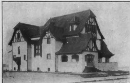
Residence of Mr. M. C. Madsen, Long Beach, L. I., covered with J-M Asbestos Stucco
