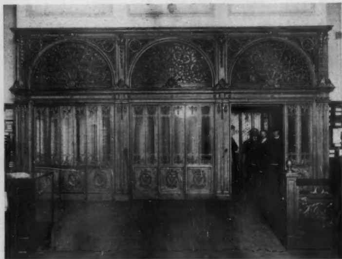
ELEVATOR ENCLOSURES, BAILLARGEON BUILDING, SEATTLE Saunders & Lawton, Architects
