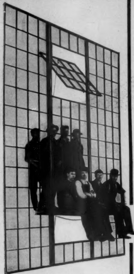
Eight Men Balanced on Ventilator Frame
