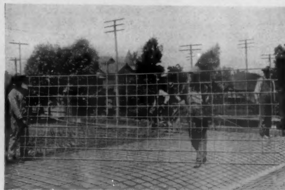
100 SQUARE FEET OF REINFORCEMENT HANDLED AS ONE BAR
