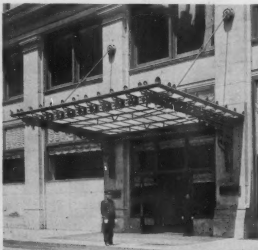
MARQUISE, McCORMICK BLDG., CHICAGO
