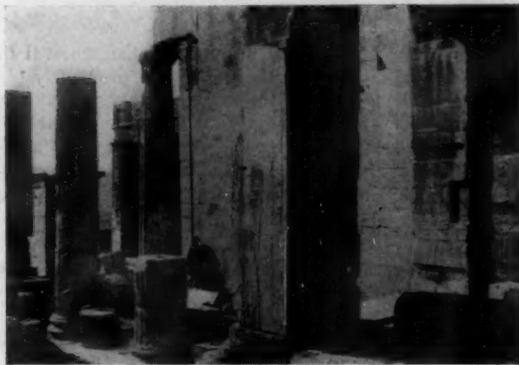
DETAIL OF INTERIOR OF GREAT HALL, SHOWING DOORS THROUGH SCREEN WALL SEPARATING EAST AND WEST PORTICOES
