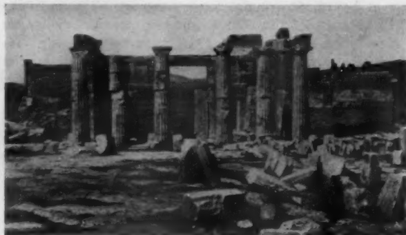
EAST FRONT BEFORE RESTORATION PHOTOGRAPH TAKEN IN 1908 Note the "ears" projecting from the stones of the north and south wing walls—evidence of the incomplete character of the work.
