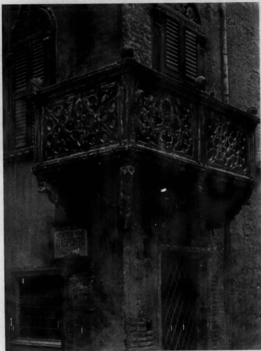
BALCONY, PALAZZO FRANCHINI, VERONA, ITALY
