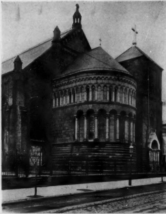
THE APSE, ST. CLEMENT'S CHURCH, PHILADELPHIA, PA., AFTER ALTERATIONS. HORACE WELLS SELLERS, ARCHITECT
