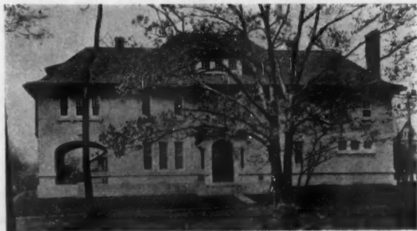
House built of terra cotta hollow tile blocks, with plaster finish at Orange, N. J. Dillon, McLellan & Beadle, Architects (From The Brickbuilder .)
