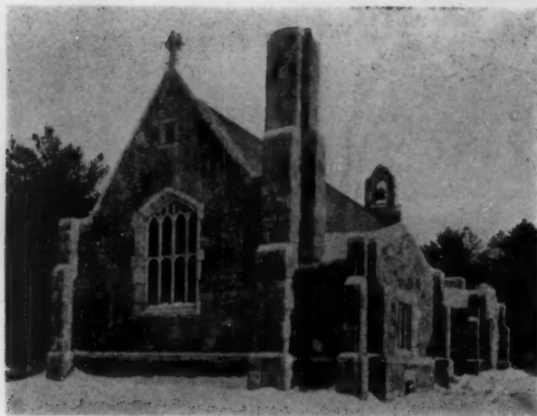
Chapel at Hudson, N. Y. Hubert G. Ripley, Architect (From The Architectural Review .)
