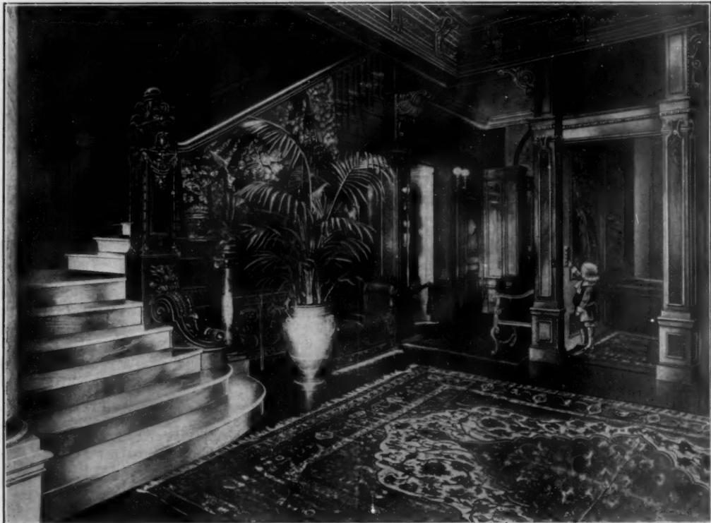
ENTRANCE TO OTIS RESIDENCE ELEVATOR
