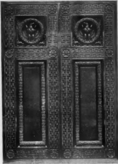
BRONZE ENTRANCE DOORS ROCHESTER TRUST AND SAFE DEPOSIT CO. YORK & SAWYER, ARCHITECTS.
