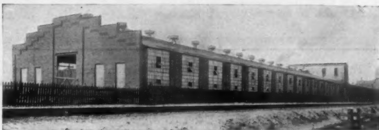
Addition to the Dodge Manufacturing Company's East Foundry at Mishawaka, Ind. A Building 360 feet long and 80 wide. Equipped in most modern fashion with Detroit-Fenestra.
