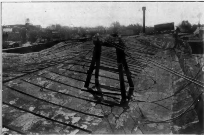
This photograph shows the "TARGET AND ARROW" tin roof of the department store of George B. Davis & Company, No. 3930 Lancaster Avenue, Philadelphia, after a fire that destroyed this building on April 24, 1910.
