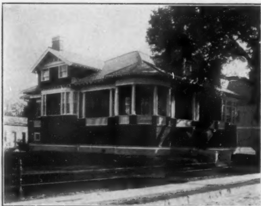
Residence of Mrs. E. M. Johnson Covered with Rising and Nelson Slate Co.'s Sea Green Slate Crosby & Henkel, Architects New Orleans, La. Jordy Bros. Slate Co., Roofers
