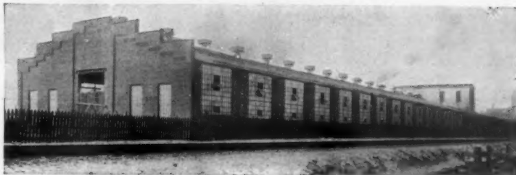
Addition to the Dodge Manufacturing Company's East Foundry at Mishawak, Ind. A Building 360 feet long and 80 wide. Equipped in most modern fashion with Detroit-Fenestra.
