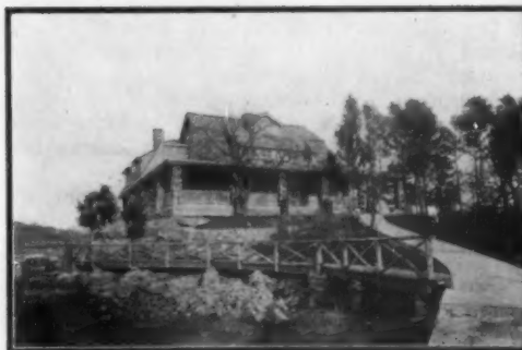
Asbestos Century Shingle Roof—Residence of Mrs. H. J. Lewis, Stony Creek, Conn. Architect and Contractor, Warren R. Briggs, Bridgeport, Conn.
