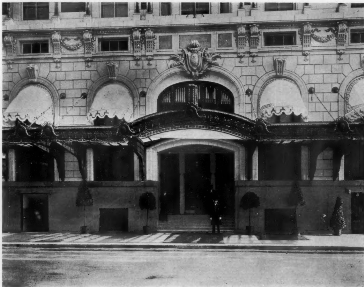
ENTRANCE ON HUBBARD PLACE
