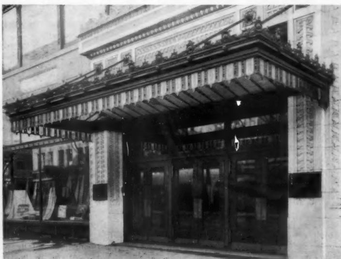
CANOPY, BAILLARGEON BUILDING, SEATTLE Saunders & Lawton, Architects
