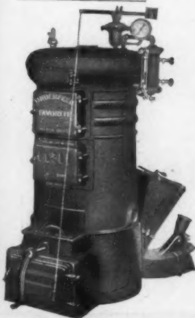
This illustration shows the Underfeed Boiler.
