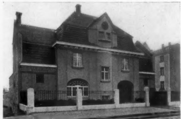
CONCRETE AND WROUGHT IRON FENCE
