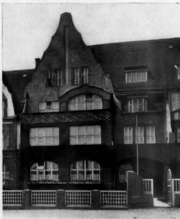
FENCE AND BASEMENT WITH THE SAME SURFACE TREATMENT
