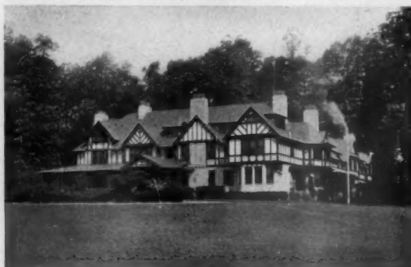
Residence of James McCrea, Ardmore, Pa. Bailey & Bassett, Architects (From The Western Architect .)
