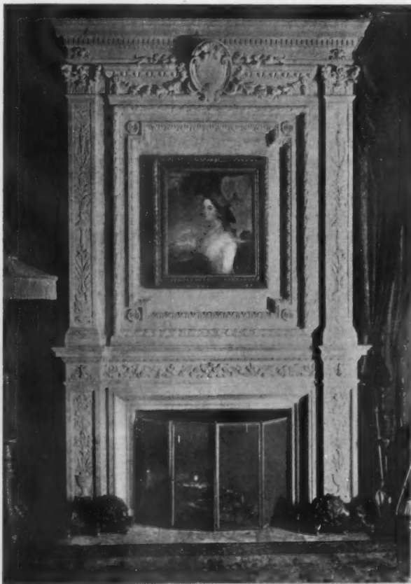
No. 1 East Seventy-fifth Street; Dining Room Mantel. Jas. Gamble Rogers, Architect
