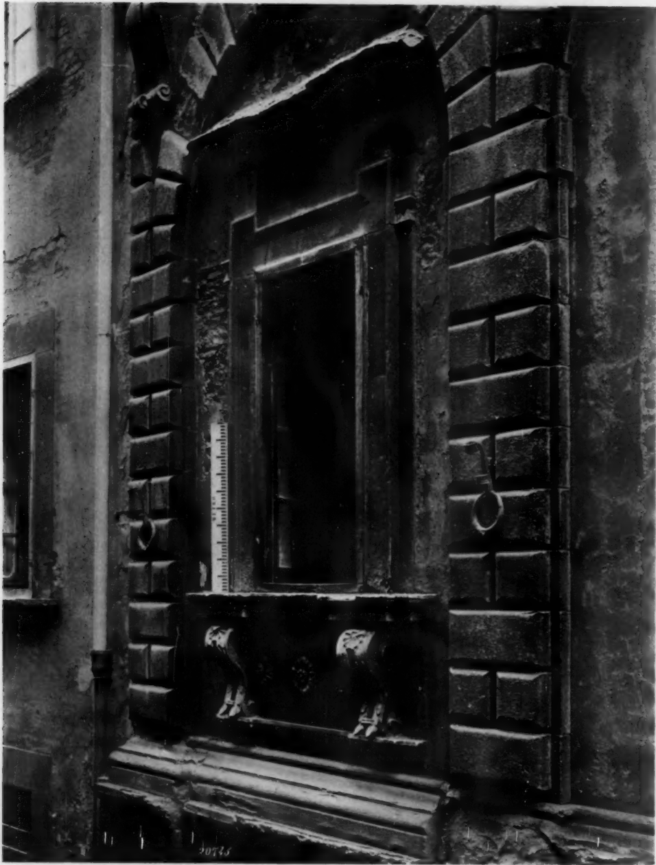
DETAIL OF WINDOW, PALAZZO MANCINI, CORTONA, ITALY.
