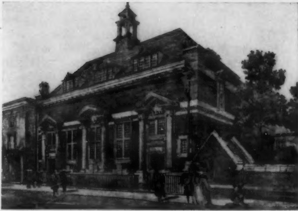
CENTRAL LIBRARY, FULHAM, ENGLAND HENRY T. HARE, ARCHITECT
