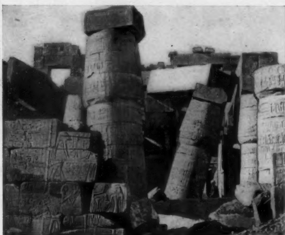
EFFECT OF THE FLOODS OF THE NILE UPON INSUFFICIENT FOUNDATIONS OF THE GREAT HYPOSTYLE HALL AT KARNAK
