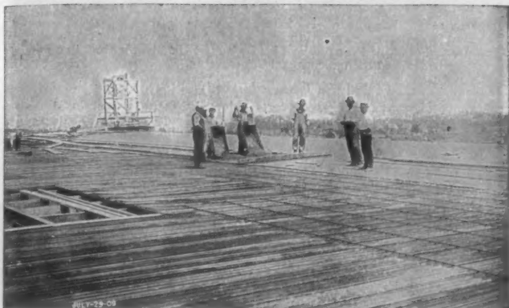
Hy-Rib Roofs for Packard Motor Car Co., Detroit
