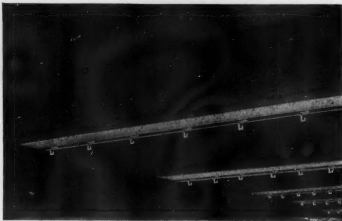
DETAIL OF CONCRETE BEAMS SHOWING REGULAR SPACING OF WHITE INTEGRAL FURRING HANGERS.
