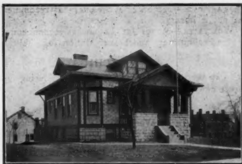
Asbestos "Century" Shingle Roof and Sheathing—Residence of W. E. Crawford, Evanston, Cincinnati, O., Fasse & Reed, Cincinnati, Architects: Bryen, Vane & Anderson, Cincinnati, Contractors
