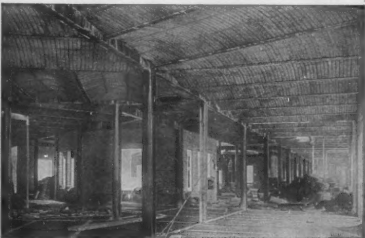
Hy-Rib Floors for St. Mary's Hospital, Milwaukee
