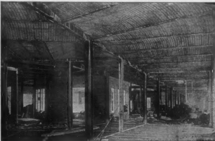
Hy-Rib Floors for St. Mary's Hospital, Milwaukee
