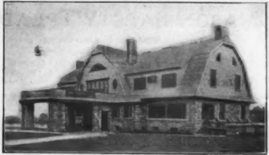
COUNTRY RESIDENCE OF HON. SETH LOW, BEDFORD STATION, N. Y. Floors deadened with Peerless Brand and side walls above first story and portions of roof insulated with Neptune Brand of Keystone Hair Insulator . Grosvenor Atterbury, Architect, New York.
