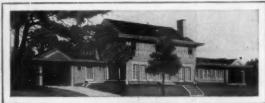
Residence of Gen. H. O. Corbin. D. H. Burnham Co., Architects.
