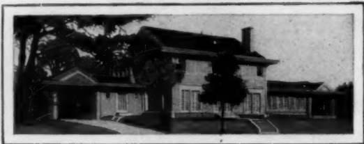
Residence of Gen. H. O. Corbin. D. H. Burnham Co., Architects.
