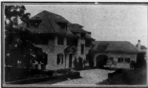
House of Mr. Rockwell Kent, Tarrytown, N. Y. Ewing and Chappell, Architects
