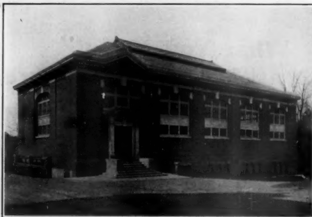
Gymnasium, Georgetown University, Washington, D. C. Ewing & Chappell, Architects
