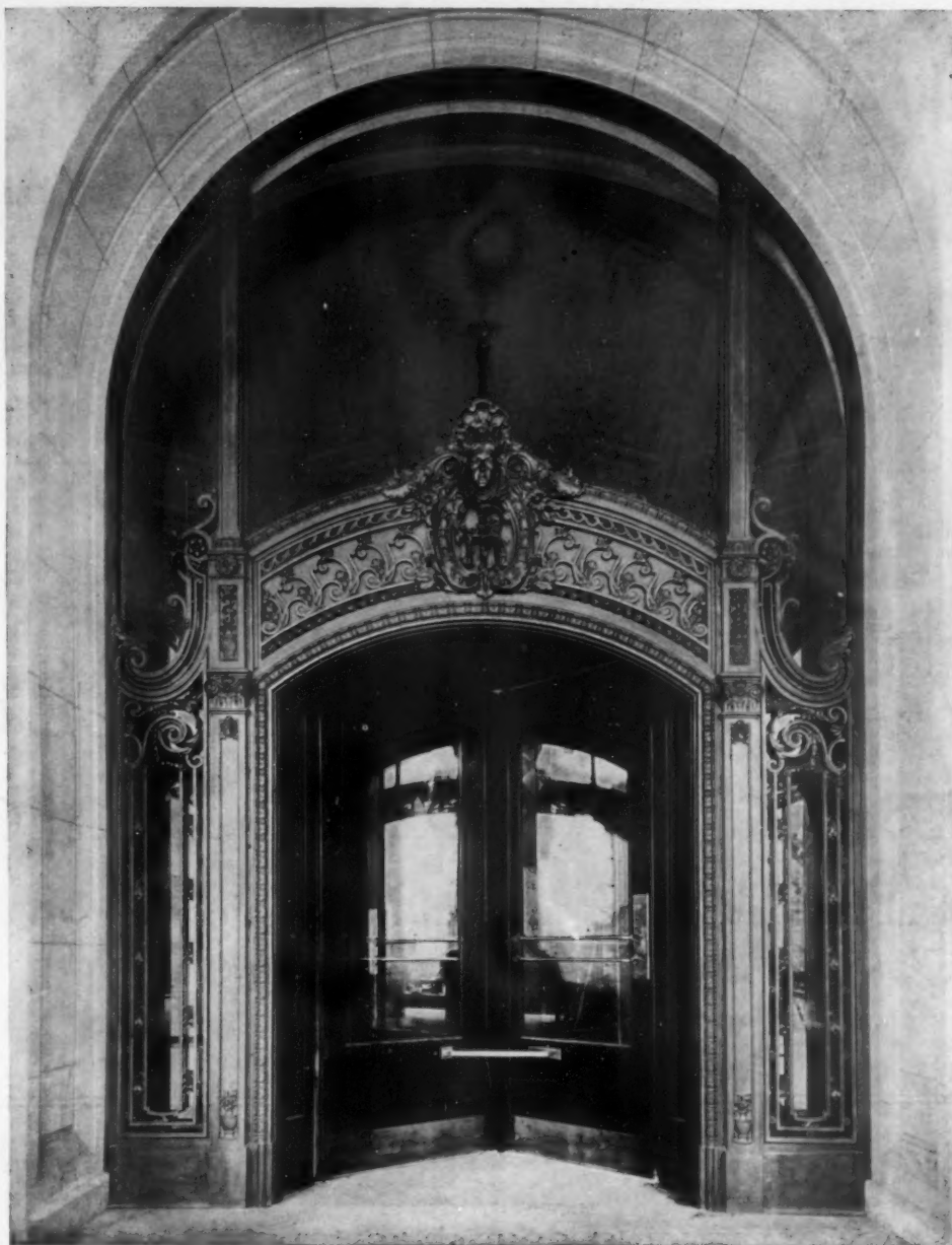
ENTRANCE, PALACE HOTEL, SAN FRANCISCO, TROWBRIDGE & LIVINGSTON, ARCHITECTS
