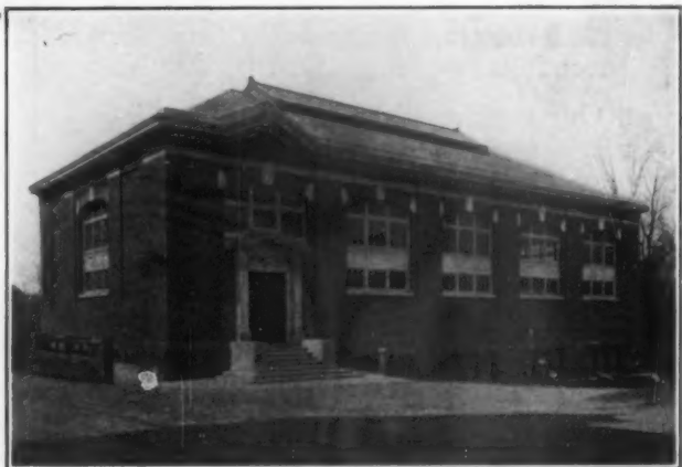
Gymnasium, Georgetown University, Washington, D. C. Ewing & Chappell, Architects
