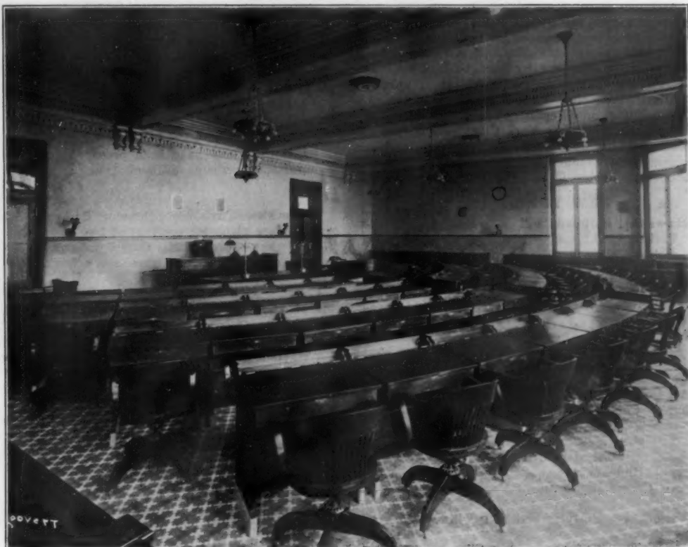
COUNTY COURT ROOM NEW SHELBY COUNTY COURT HOUSE
