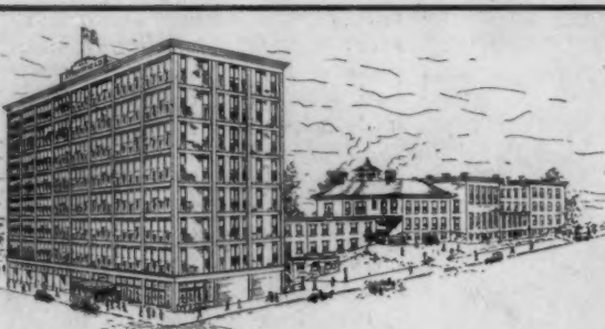
The Stratfield Hotel, Bridgeport, Conn. Berger Prong Lock Studs and B. B. Expanded Metal Lath used. Also Berger Raydiant Sidewalk Lights.
