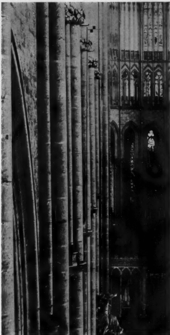
FIG. 6. AMIENS CATHEDRAL. NORTH SIDE, LOOKING EAST Plumb on third pier from crossing, showing the pier as perpendicular below the arcade capital and the vaulting shaft as deflected outward above the arcade capital. (One of 12 similar details.) Surveyor's disk (8" x 10") on the plane of measurement above the carved stringcourse; giving, by compass test, 4 inches deflection between the capital and the stringcourse. The inclination of the entire vaulting-shaft is 8-9 inches. Compare plate 10.
