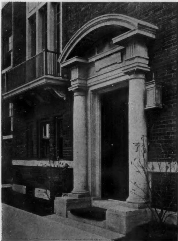
Entrance Detail, Residence of C. H. Hutchins, Chicago, Ill. Horatio R. Wilson & Co., Architects (From The Western Architect )
