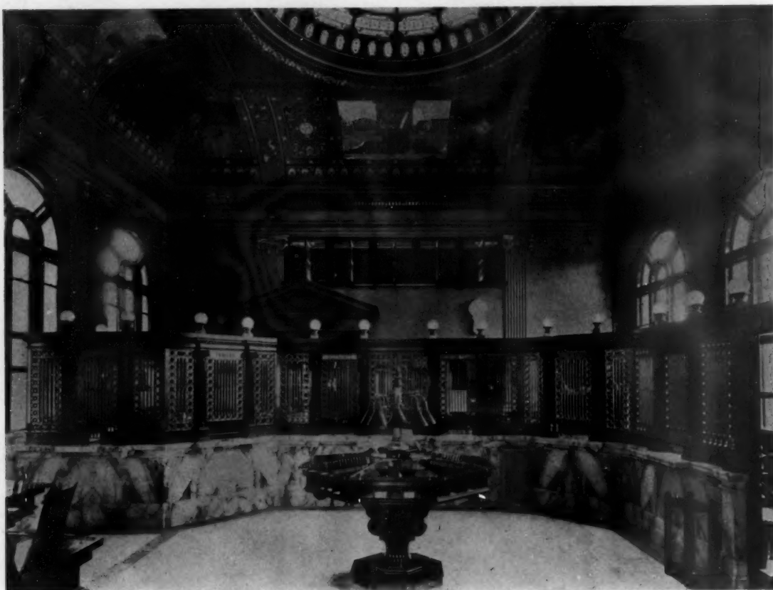
BANKING ROOM, FROM ENTRANCE
