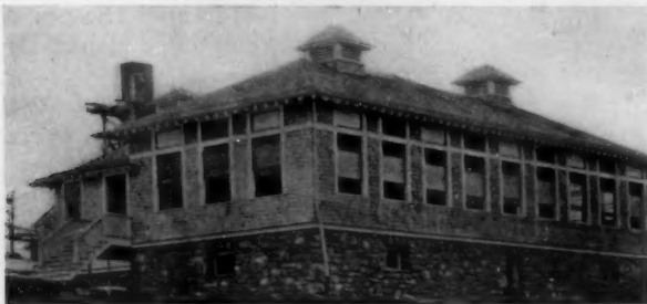
OTISVILLE SANATORIUM, NEW YORK. ADMINISTRATION BUILDING FOR MEN'S UNIT. COST, $35,000. DESIGNS OF THE DEPARTMENT OF HEALTH. JOHN V. VAN PELT, ARCHITECT
