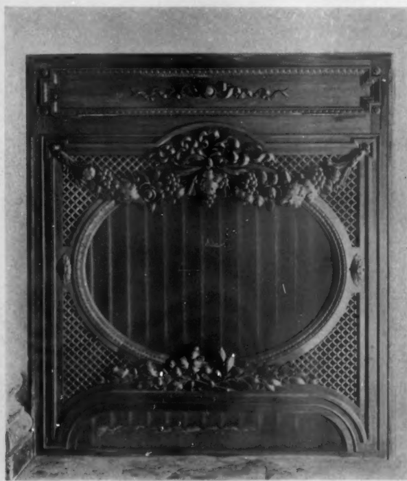
THE "ACRAN" DESIGNED TO CONCEAL THE RADIATORS SET IN THE WALL.
