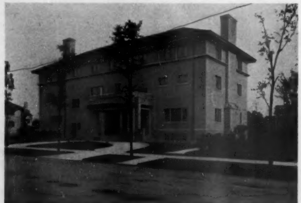
A House at Chicago, Ill. Nimmons & Fellows, Architects
