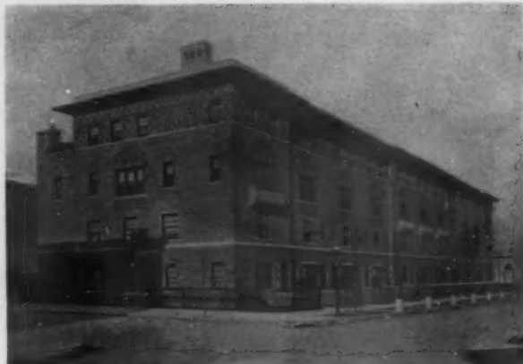
Kinko Duplex Apartment, Brooklyn, N. Y. Mann & Macneille, Architects
