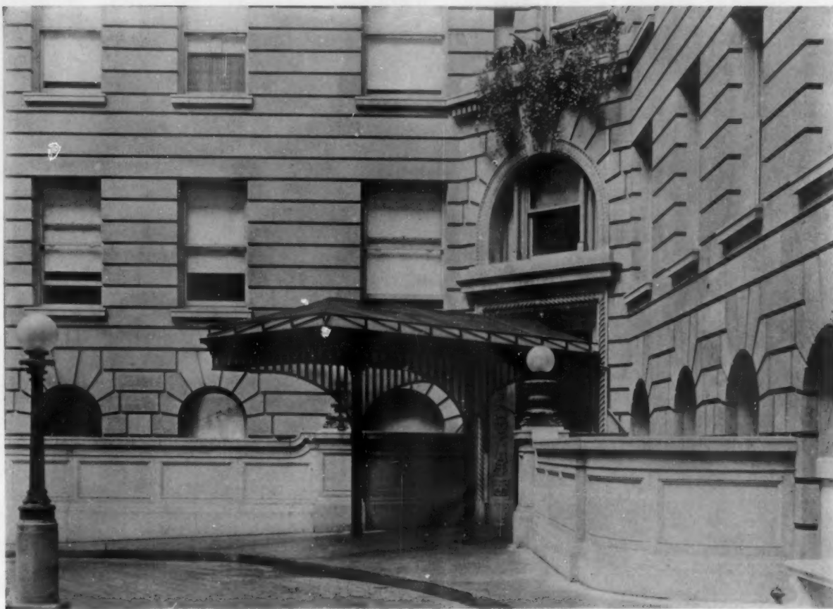
DETAIL OF DOORWAY IN COURTYARD
