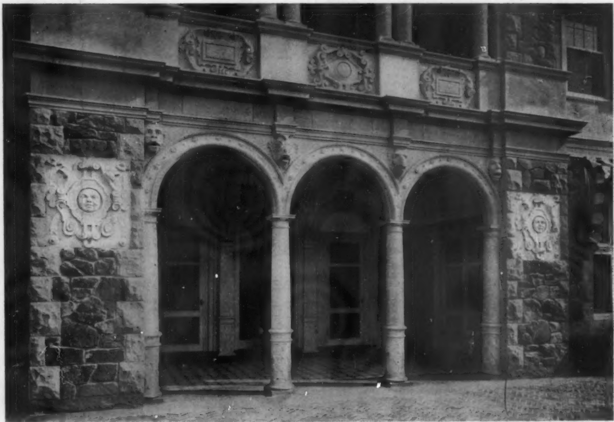
DETAIL OF LOGGIA
