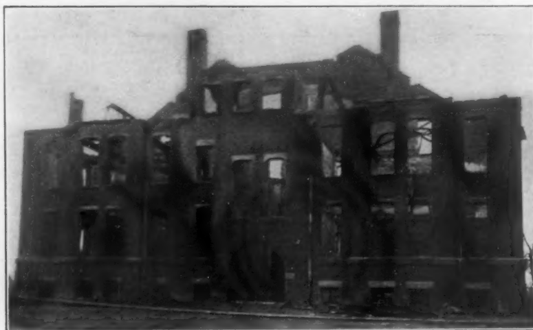
RUINS LAKEVIEW SCHOOL, COLLINWOOD, OHIO
