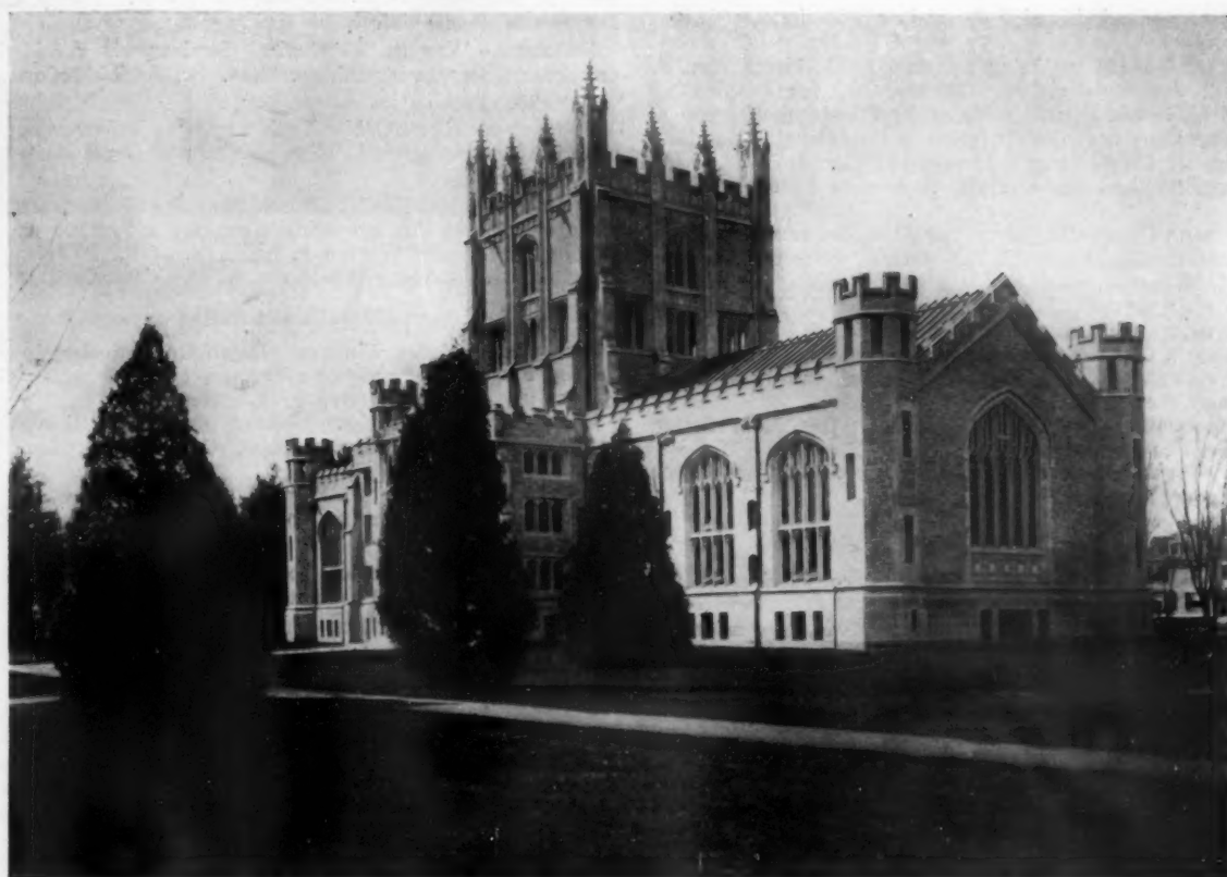
Allen & Collens Architects Boston
