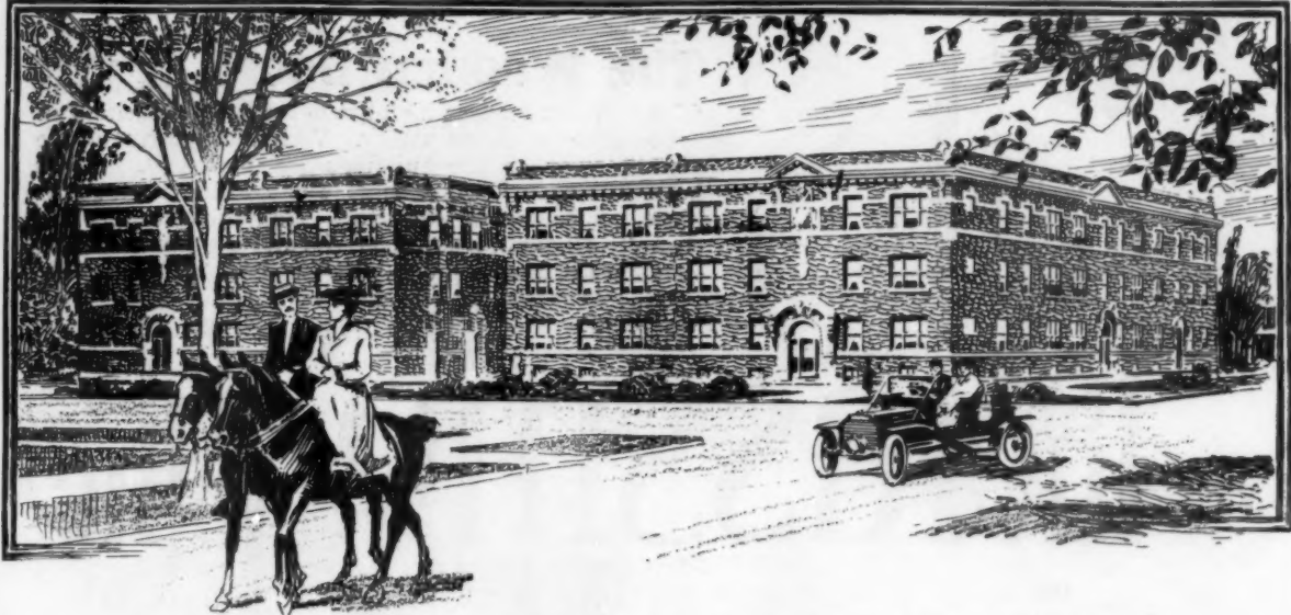
The beautiful Pueblo Apartments, Chicago, Ill. (E. J. Ohrenstein, architect), are heated by three Kewanee Firebox Boilers.
