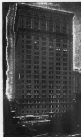
U. S. Express Building, New York. Clinton & Russell, Architects
