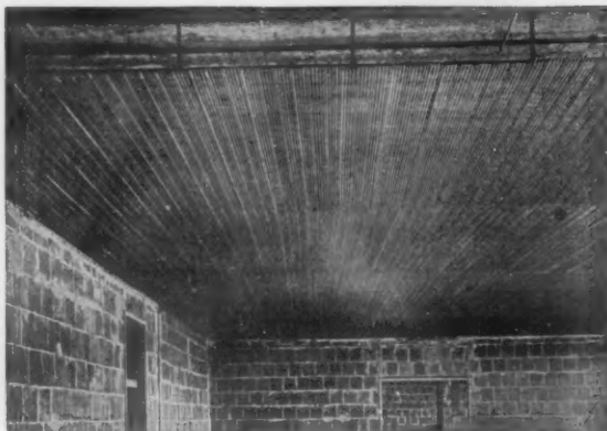
Hy-Rib Ceiling, Mt. St. Joseph Academy, Buffalo, N. Y. A. A. Po-t, Architect. John Lannen, Contractor
