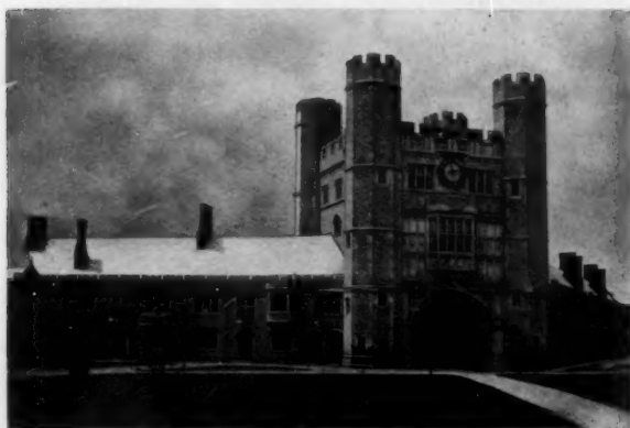
Princeton University Chemical Laboratory covered with J-M Asbestos Roofing
