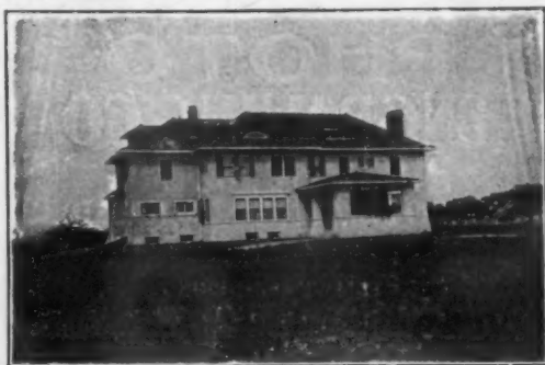
Residence of Dr. H. M. Pollock, Superintendent Norwich State Hospital, Norwich, Conn., Oudworth & Woodworth, Architects.
