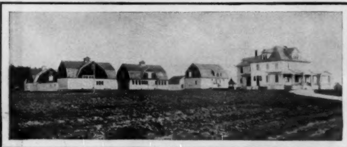
"Fairview" Estate of Mr. Chas. H. Foote, Burlington, Vt. Frank Lyman Austin, Arch.
