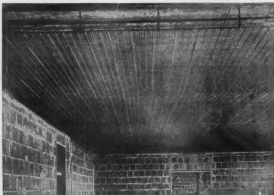
Hy-Rib Ceiling, Mt. St. Joseph Academy, Buffalo, N. Y. A. A. Post, Architect. John Lannen, Contractor.
