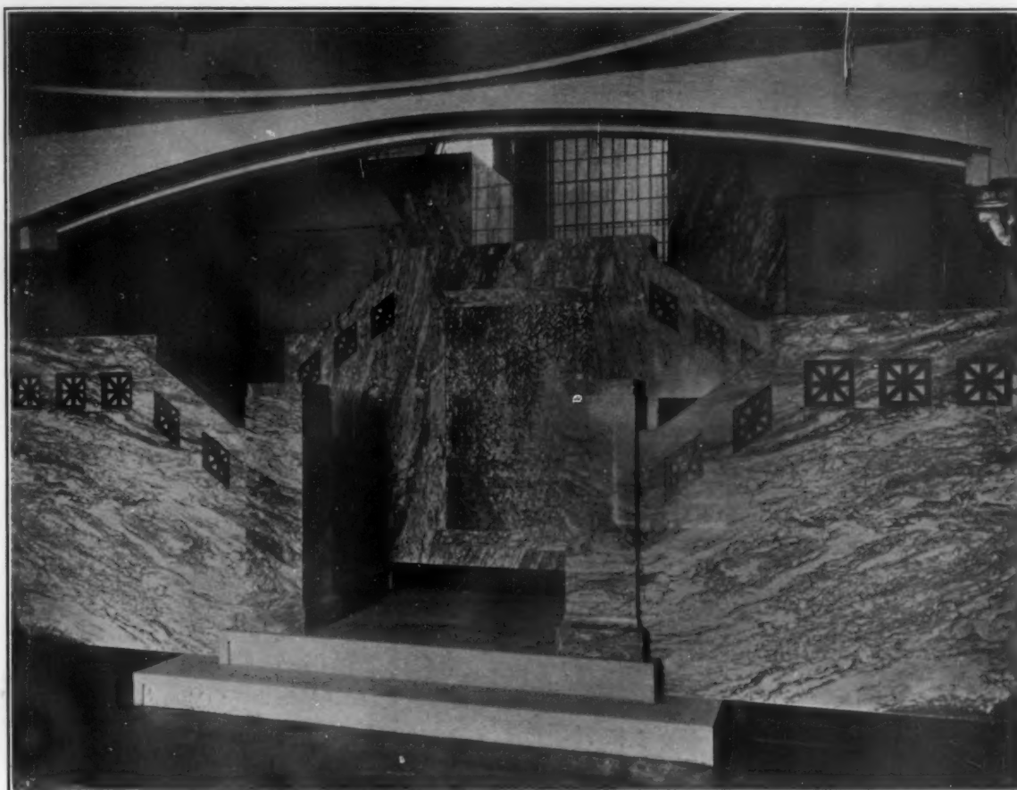
MARBLE STAIRWAY RESIDENCE OF MR. J. W. THOMPSON, ST. LOUIS
