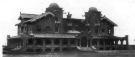
NORTH SIDE INN, JEROME, IDAHO Bostwick Steel Lath used in the construction.
