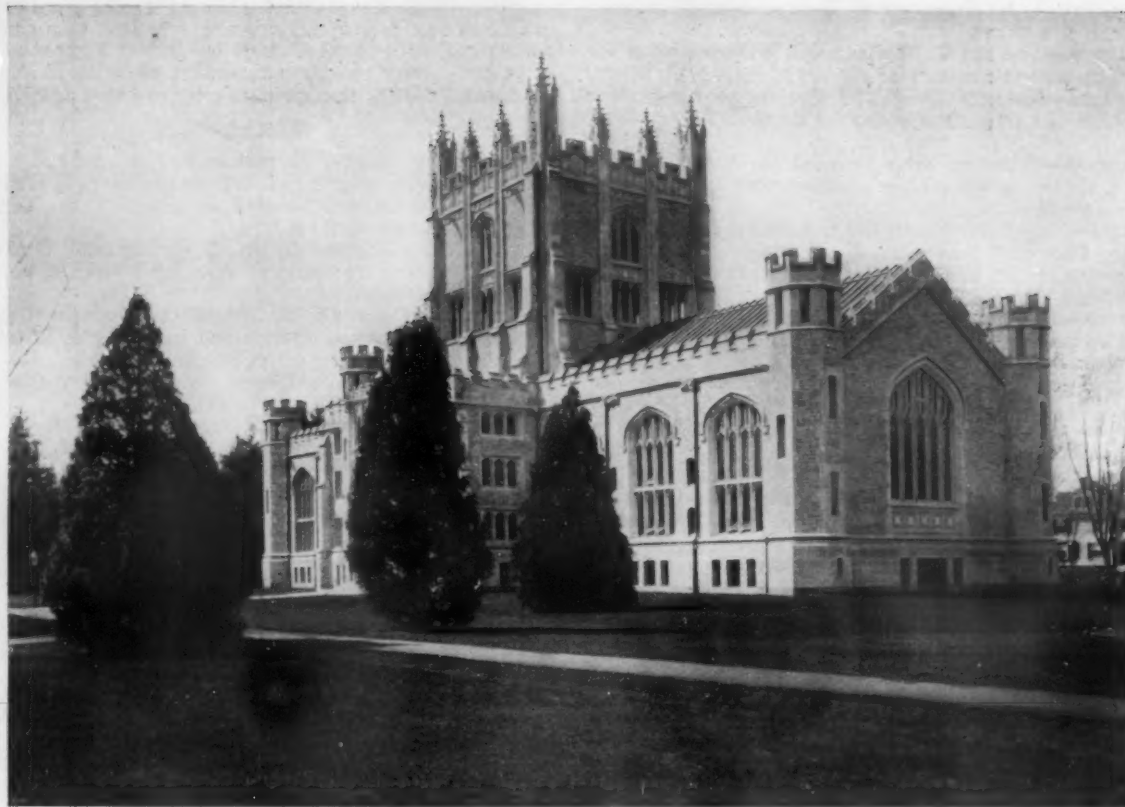
Allen & Collens Architects Boston
