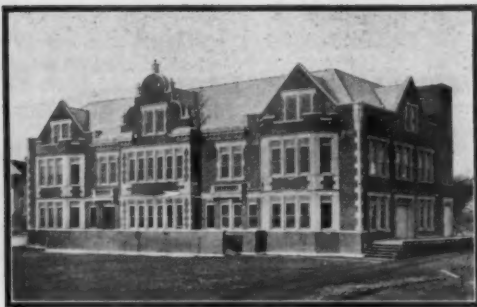
Asbestos "Century" Shingle Roof—Office Building of Wills & Baumer Co., Syracuse, N. Y.; Merritt C. Conway, Syracuse, Architect
