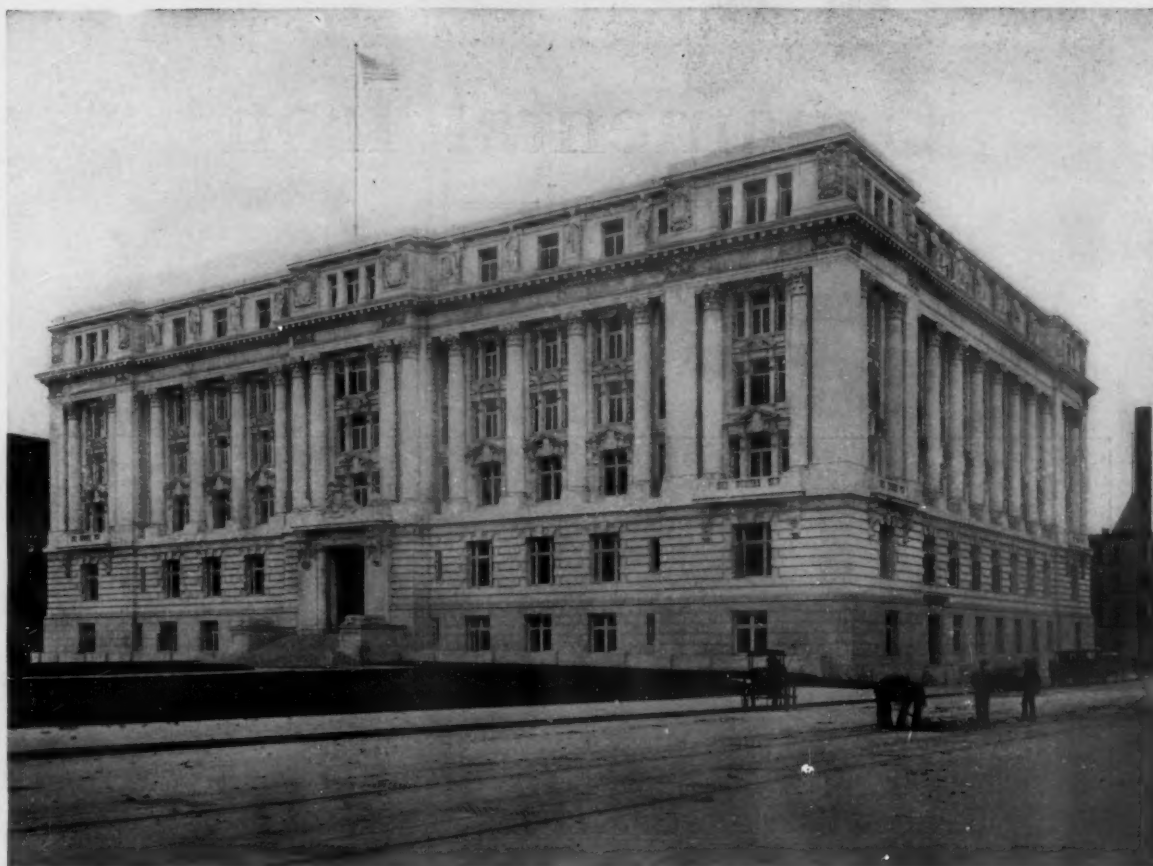
MUNICIPAL BUILDING WASHINGTON, D. C.
