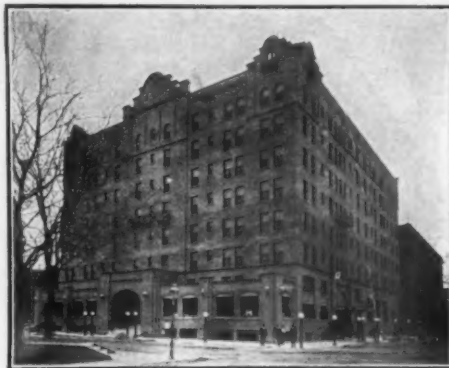
St. Anthony Hotel, San Antonio, Texas. Berger Prong Lock Studs installed. Architect, J. Flood Walker
