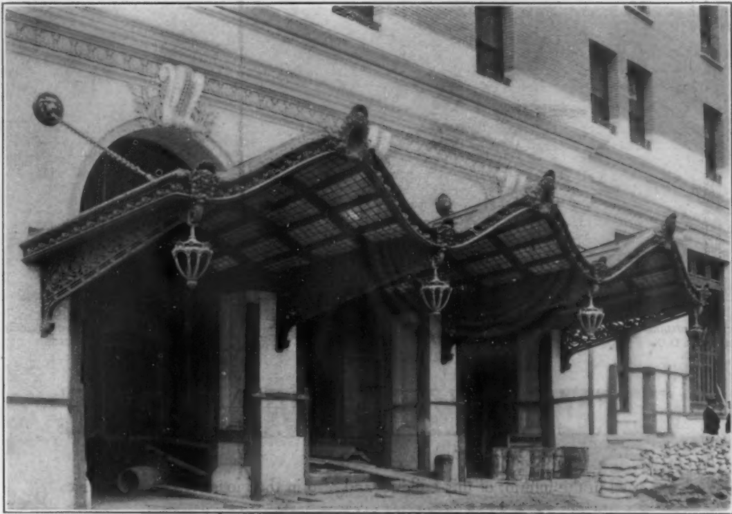
MARQUISE, PALACE HOTEL, SAN FRANCISCO, CAL. TROWBRIDGE & LIVINGSTONE, ARCHITECTS
