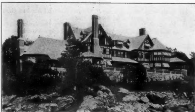
The Eben G. Jordan Summer Home, West Manchester, Mass. Wheelwright & Haven, Architects. NEPONSET insulates this residence.
