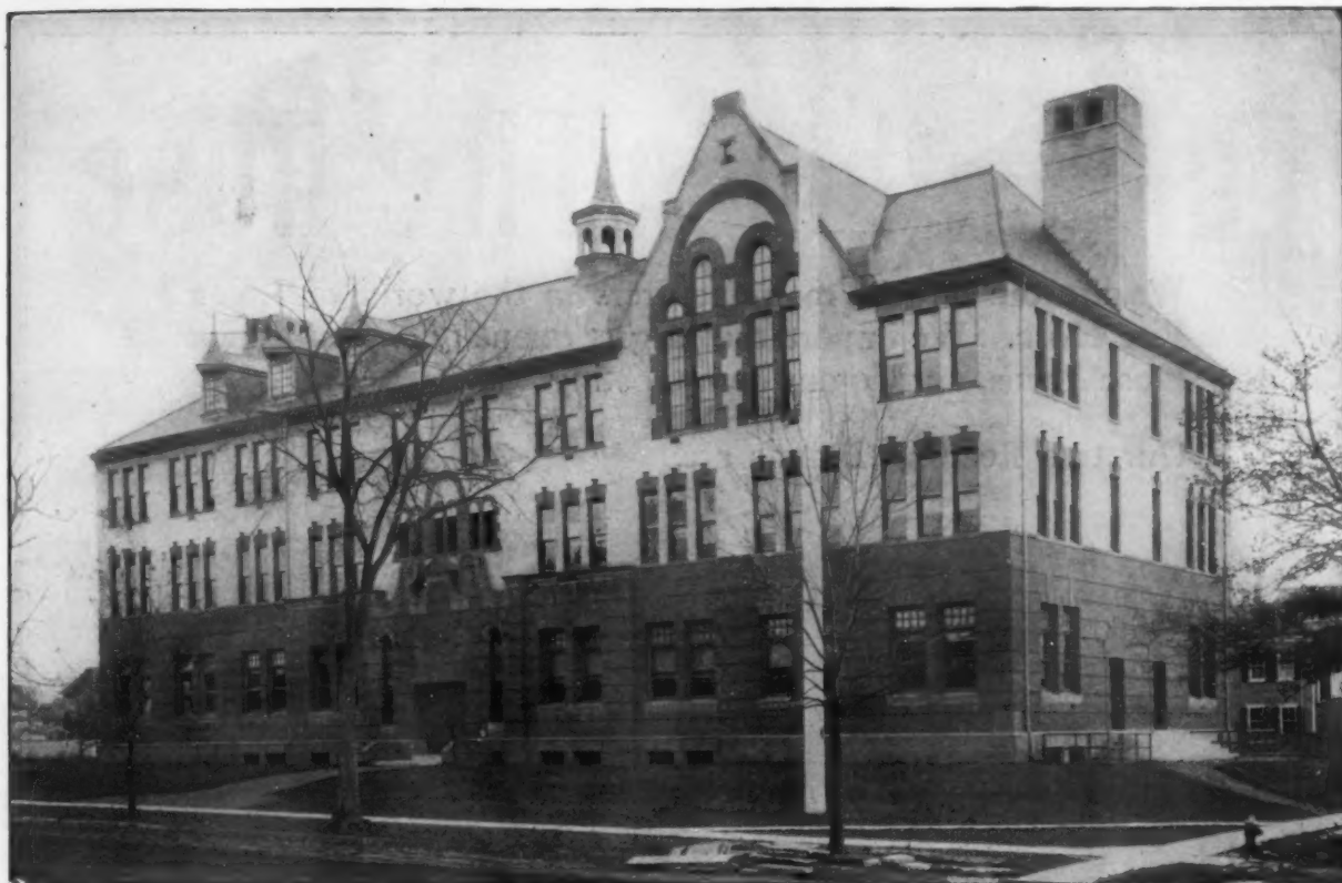
High School, Jamaica, L. I., N. Y. Deadened with Cabot's Deafening Quilt. W. B. Tubby, Architect, New York City.
