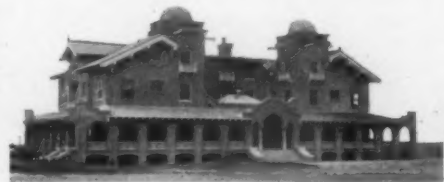
NORTH SIDE INN, JEROME, IDAHO Bostwick Steel Lath used in the construction.
