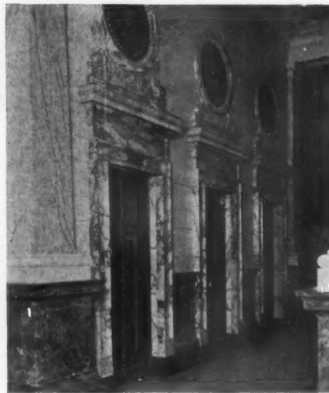
Marble Entrance to Elevators in "Tower" (Twenty-fourth Street) Metropolitan Life Insurance Co. Building
