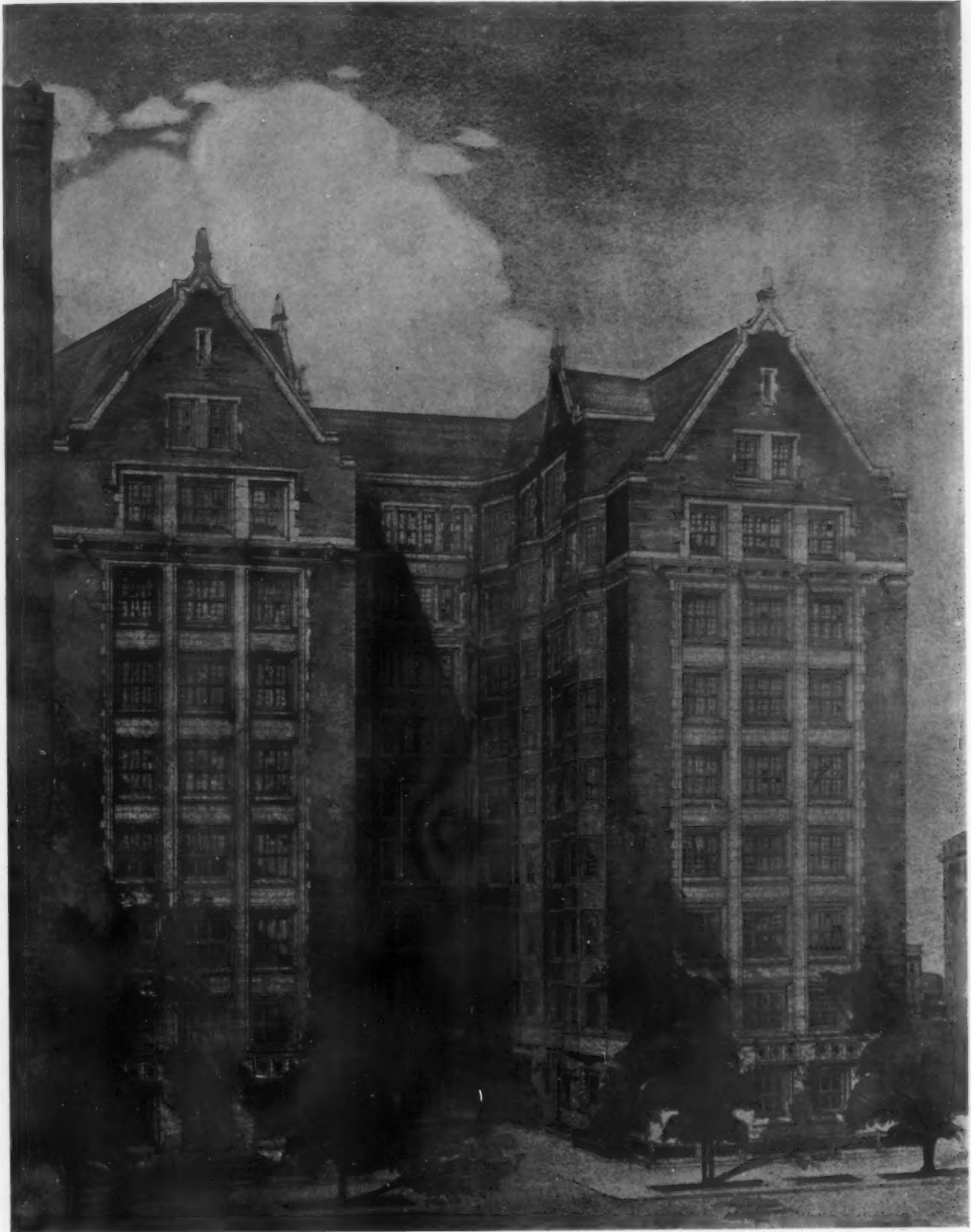
THE BRITANNIA APARTMENTS CATHEDRAL PARKWAY, NEW YORK
