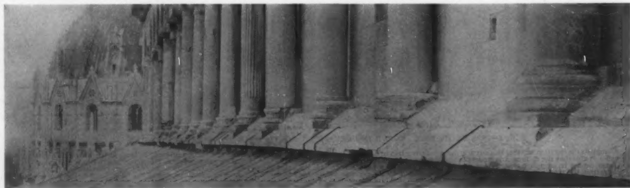
FIG. 7—PISA CATHEDRAL. CURVE OR BEND, IN ELEVATION OF THE SOUTH CLERESTORY BASE MOULDING
