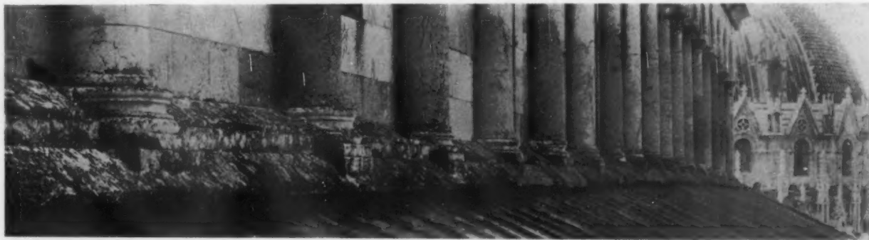
FIG. 4.—PISA CATHEDRAL. CURVE IN ELEVATION OF THE NORTH CLERESTORY BASE MOULDING
