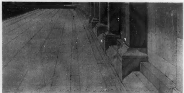
FIG. 11—PISA CATHEDRAL. CURVE IN PLAN OF THE SOUTH WALL LOOKING WEST
