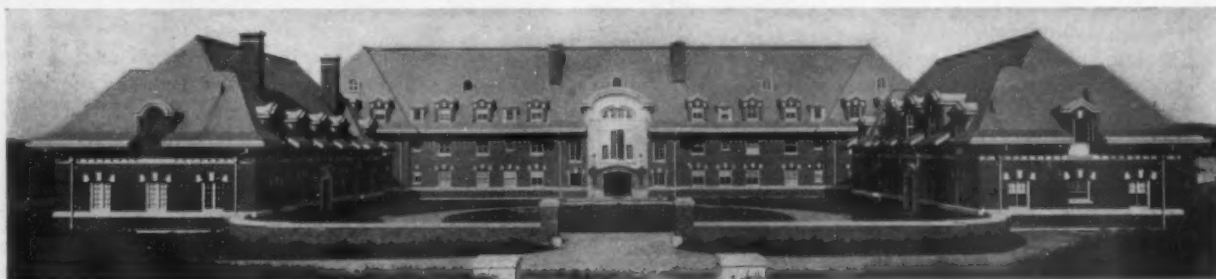
SCHOOL AT BRIAR CLIFF MANOR, N. Y.
