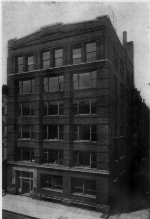
WAREHOUSE OF PARKE, DAVIS & CO., CHICAGO, ILL. MESSRS. HILL & WOLTERS DORF, ARCHITECTS
