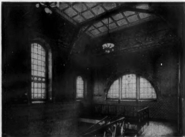
STAIRCASE AND HALL OF THE NEW PUMPING STATION COLOGNE, GERMANY HERR J. GÄRTNER, ARCHITECT
