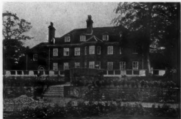
FRITHWOOD HOUSE, NORTHWOOD GARDEN FRONT
