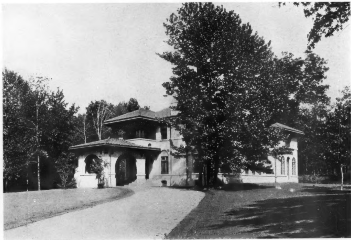
HOUSE OF DAN FELLOWS PLATT, ESQ. ENGLEWOOD, N. J.
