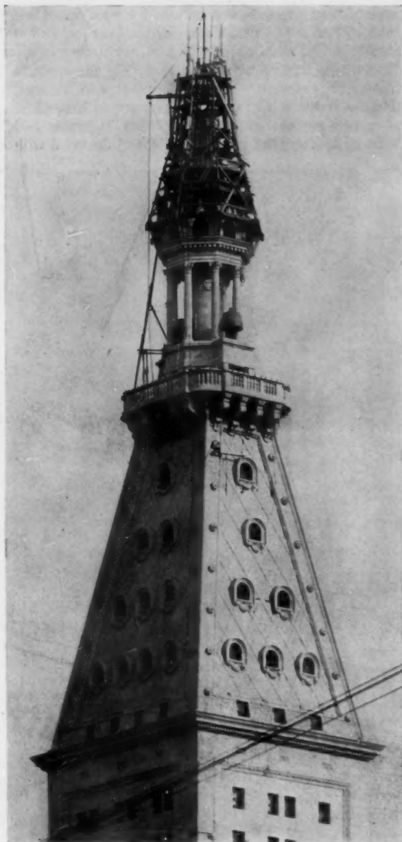
TELEPHOTO VIEW OF TOP OF TOWER DURING CONSTRUCTION
