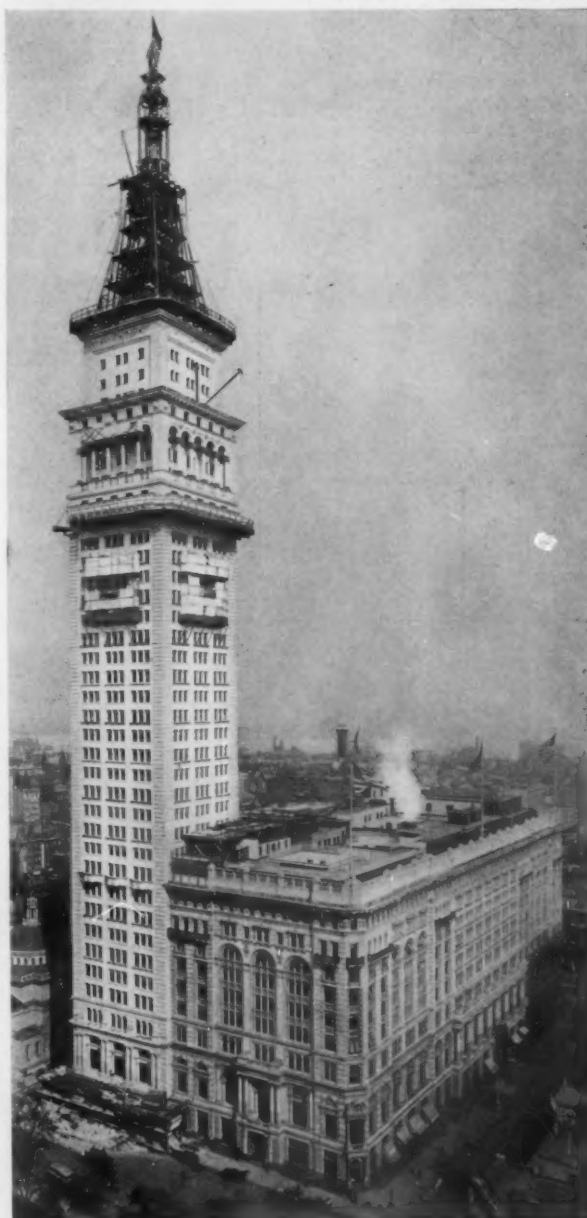
VIEW FROM SOUTHWEST DURING CONSTRUCTION
