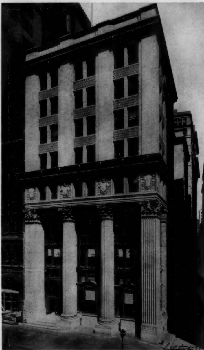
THE DOWNTOWN BUILDING, BROADWAY, NEW YORK CITY, is equipped with four
