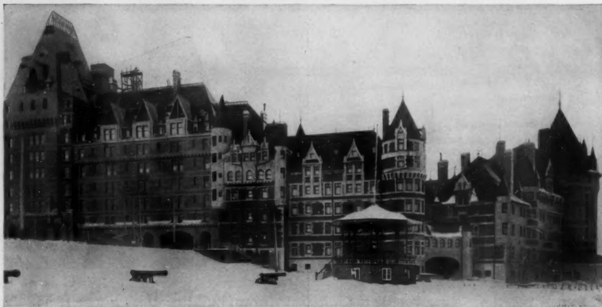
ADDITION TO CHATEAU FRONTENAC, QUEBEC, QUE.
