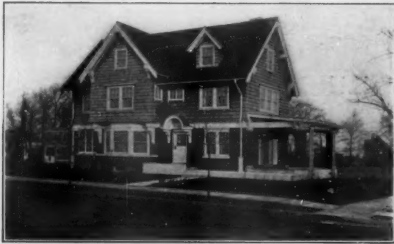
The Thomas L. Morton Residence Newark, N. J. William F. Cone, Architect
