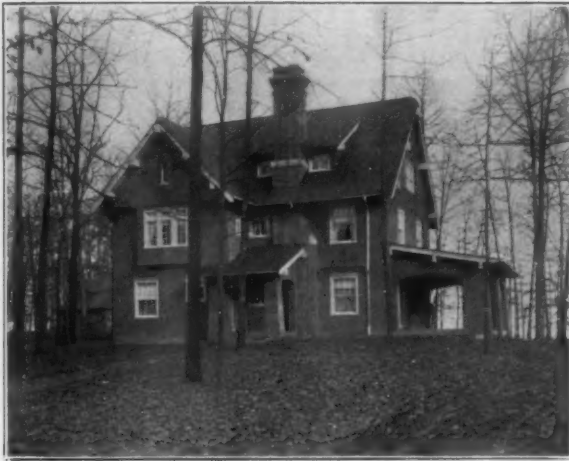
The Chas. Cluthe Residence, Glen Ridge, N. J. Insulated with NEPONSET. William F. Cone, Architect, Newark, N. J.
