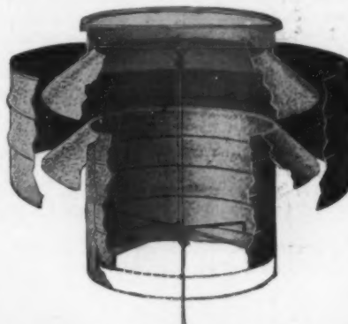
Notice Sliding Sleeve Damper. (Patented.)
