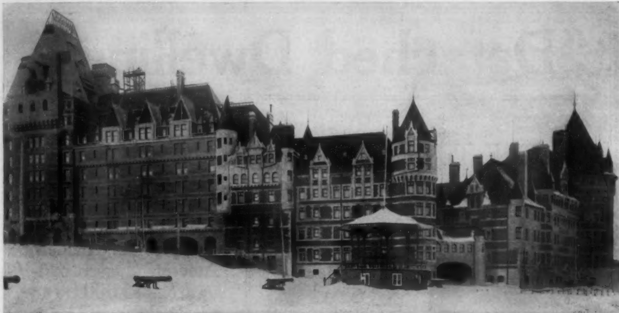
ADDITION TO CHATEAU FRONTENAC, QUEBEC, QUE.
