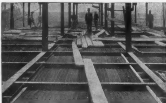
Arched Hy-Rib Floor at St. Mary's Hospital, Milwaukee, Wis. Esenwein & Johnson and J. D. Gregg, Archts. Newton Eng. Co., Contra.
