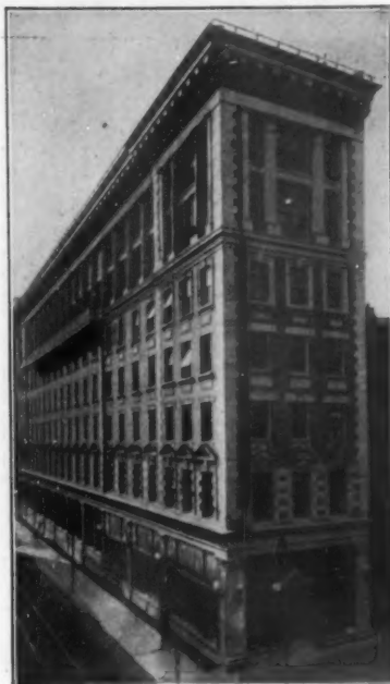
Philadelphia Electric Co. Building Architect, James T. Windrim Berger "Prong Lock" Steel Studs installed
