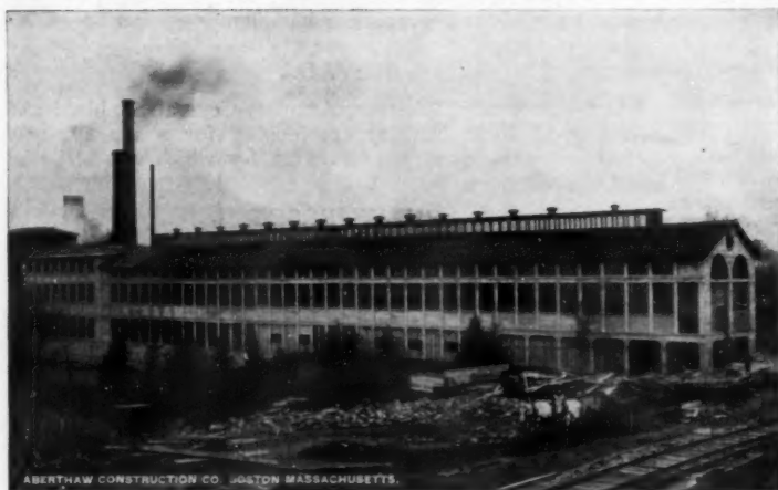
ABERTHAW CONSTRUCTION CO. BOSTON MASSACHUSETTS.
