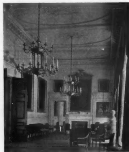
GOVERNOR'S ROOM, CITY HALL, NEW YORK RESTORATION BY GROSVENOR ATTERBURY, ARCHITECT
