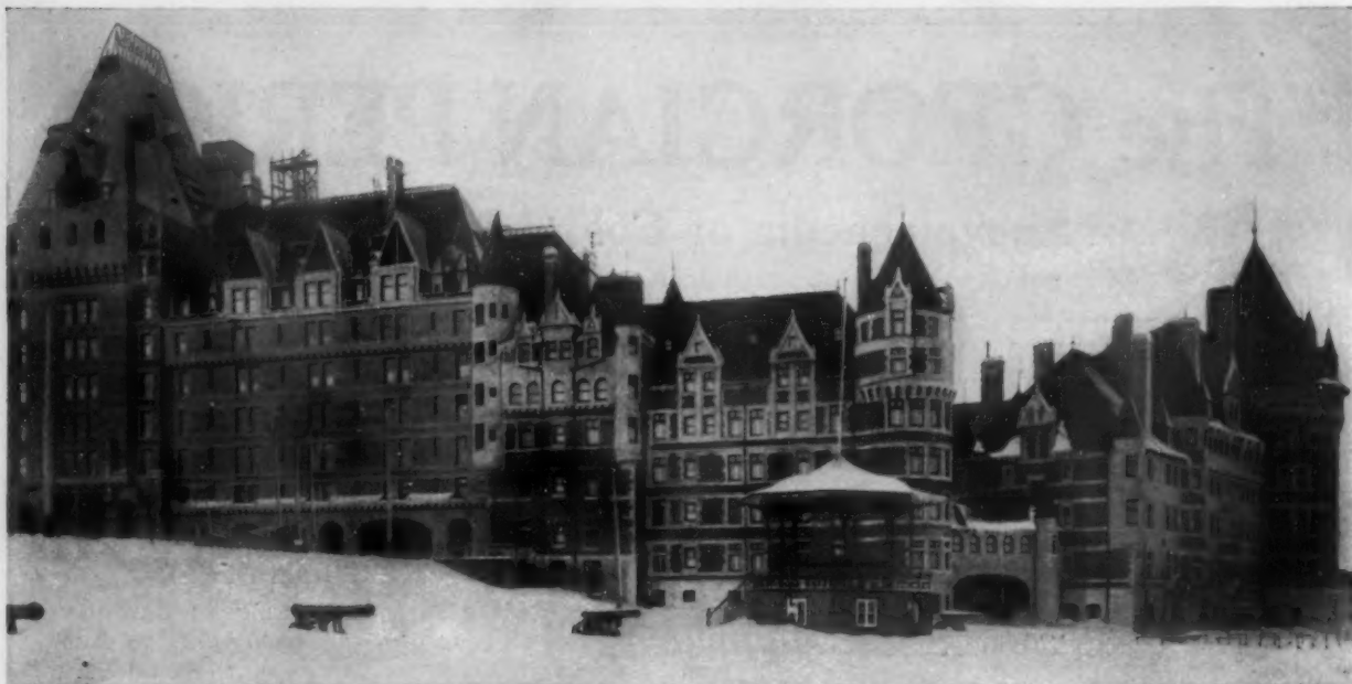
ADDITION TO CHATEAU FRONTENAC, QUEBEC, QUE.
