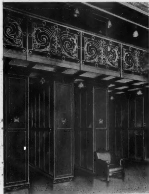
LIBRARY INTERIOR executed by ART METAL CONSTRUCTION CO. JAMESTOWN, N. Y.
