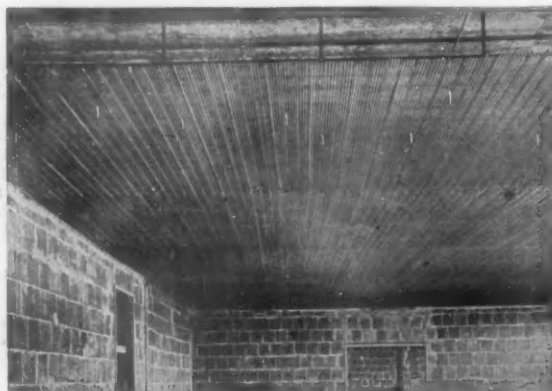
Hy-Rib Ceilings in Mount St. Joseph Academy, Buffalo, N. Y. A. A. Post, Architect. John Lannen, Contractor.
