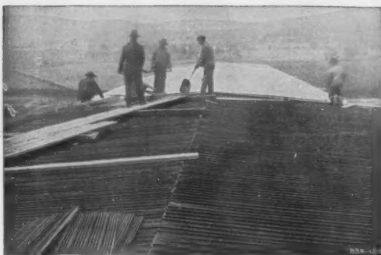
Hy-Rib Roof for American Car and Foundry Co., Berwick, Pa.
