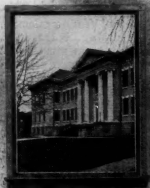
Same Building Taken Through a Window Glazed With Polished Flawless Plate Glass.
