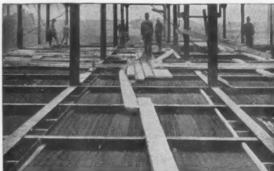
Arched Hy-Rib Floor at St. Mary's Hospital, Milwaukee, Wis. Esenwein & Johnson and J. D. Gregg, Archts. Newton Eng. Co., Contrs.
