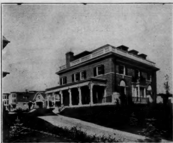
ELEGANT NEW RESIDENCE AT READING, PA. Charles F. Rabenold, Philadelphia, Pa., Architect HEATED BY TWO NO. 27 KELSEY GENERATORS
